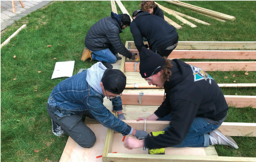
Image: Group construction work on POD I, Fall 2021
