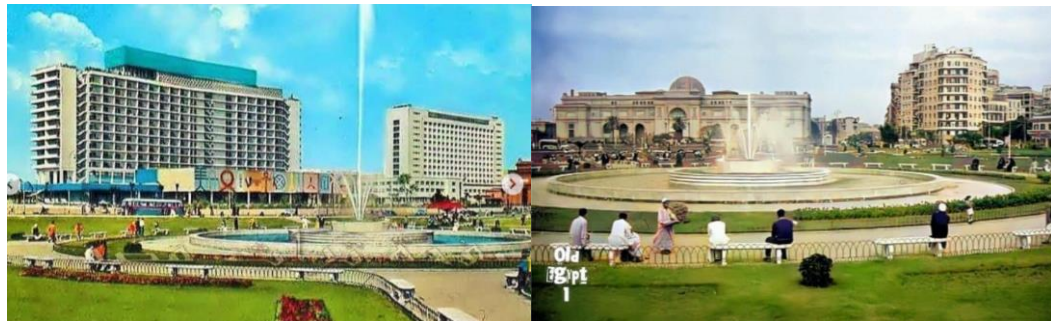
Figure 5.21 Tahrir Square fountain and park in the 1960s.
