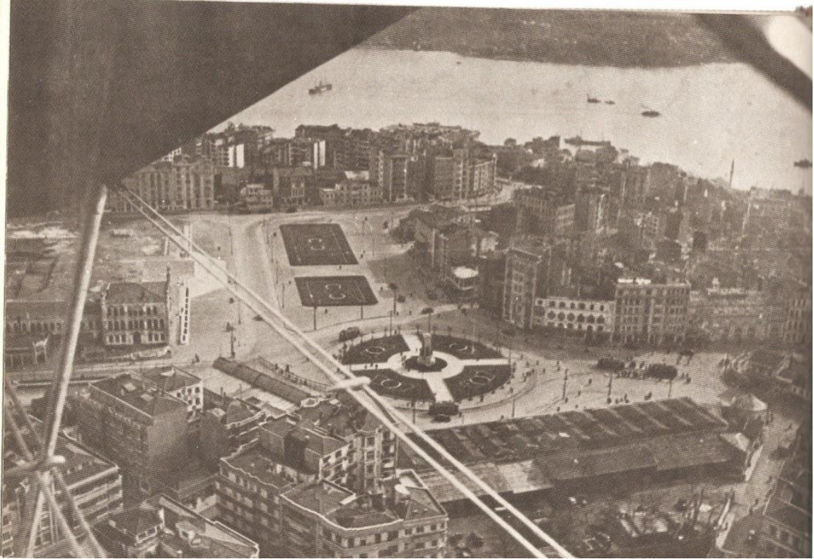
Figure 2.3 The newly regulated spaces in and around Taksim Square. The above photograph taken from an airplane shows the grand façade of the Artillery Barracks on the left side. The historical Taksim water distribution building that is located across the Monument of the Republic (at the center of the circular green area/roundabout) is below on the right. The tramway station is located at the entrance of İstiklal Street on the right-hand side of the image. Since the demolition of the barracks was not finalized when the photograph was taken, it can be argued that it dates between 1940 and 1942. Source: Çelik Gülersoy, Taksim: Bir Meydanın Hikayesi (Istanbul: 1986), 52.
