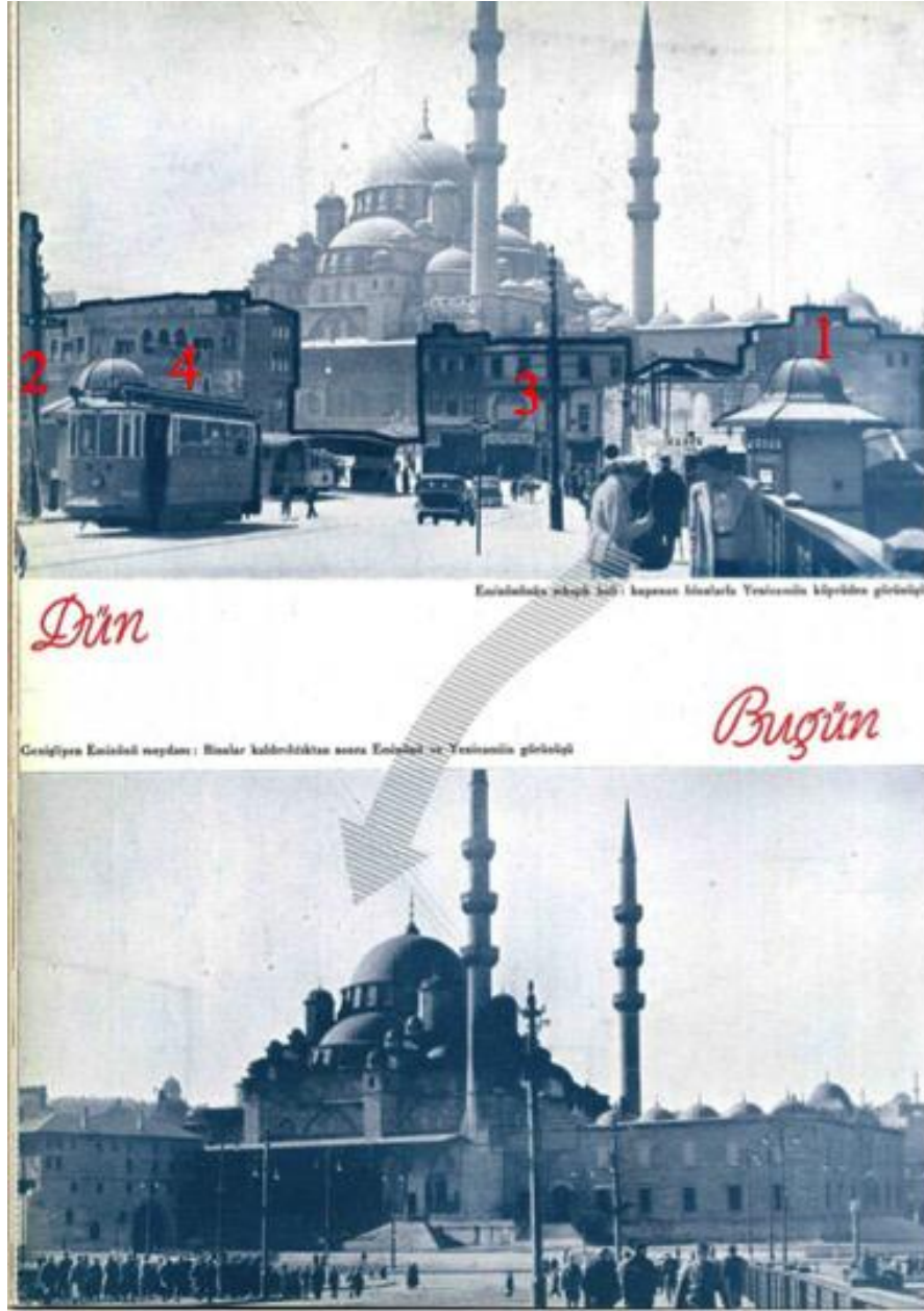
Figure 2.5 Before and after conditions of the clearance of buildings surrounding the New Mosque in Eminönü. In the first picture, the square was clustered with two- and three-story buildings. After the demolitions, the New Mosque became the main visual element that dominated and defined the broadened square. Also, the tramway station was moved, and thus, the pedestrian movement was redefined.
