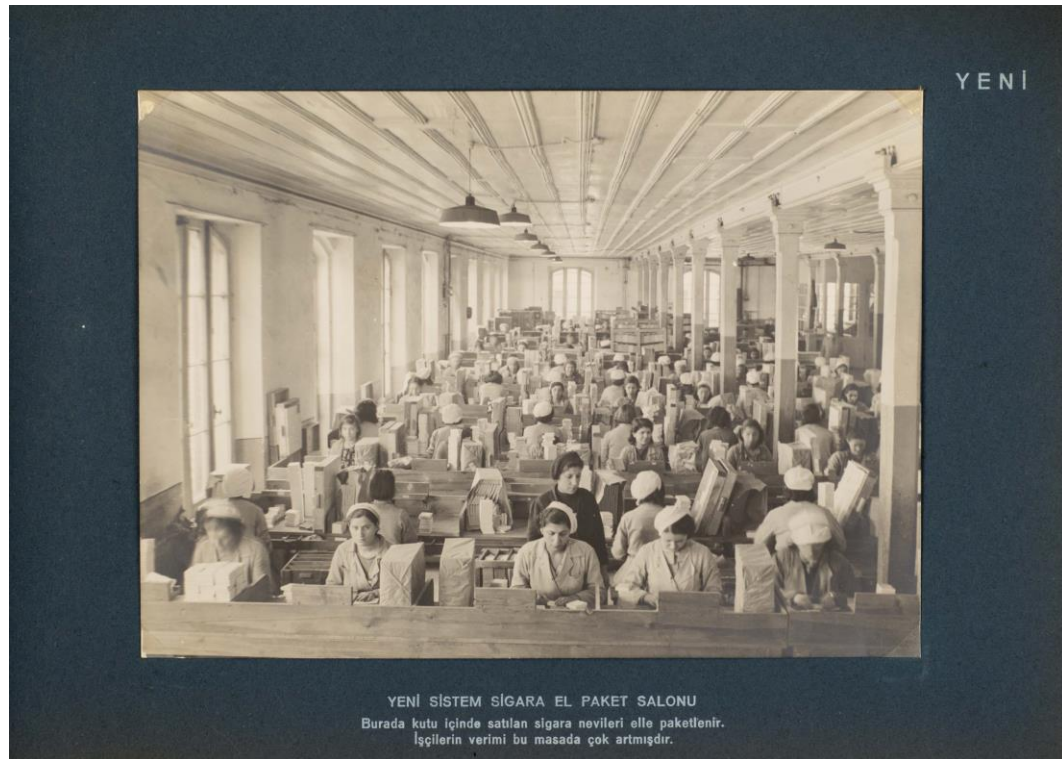
Figure 3.16 The production hall where different types of cigarettes were packed by hand. The caption states that productivity was increased with the new organization. Source: The Photograph Album of the Tobacco Monopoly Administration of the Turkish Republic, 1940, Rezan Has Museum Collection.
