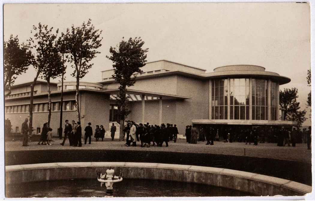
Figure 2.18 Taksim Municipality Gazino. The most striking part of the design was the double-height semicircular glass wall projecting towards the park. There was a pool by the entrance which is visible at the bottom of the image. People seem to leave the gazino in groups consist of both women and men. Since it was still daytime, it can be imagined that they attended a tea party at the gazino .
