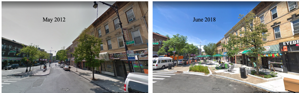
Figure A.3 Before and after images of 71 st Avenue Plaza. Source: Google Earth.
