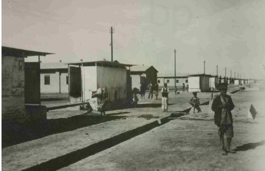
Figure 4.20 A view of a Back-Service Alley in the New Workmen’s Village, circa 1935. The alleys served as infrastructural conduits accommodating the sanitary facilities, such as surface drainage, water hydrants, bathing cubicles, and dry latrines.
