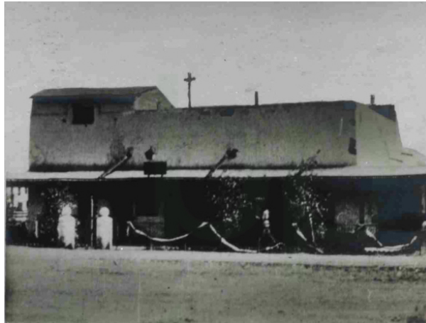
Figure 3.36 Abadan Police Station, circa 1921. Constructed based on the second-class colonial buildings, the Police Station represented the industrial vernacular style in Abadan in the post-war years.
