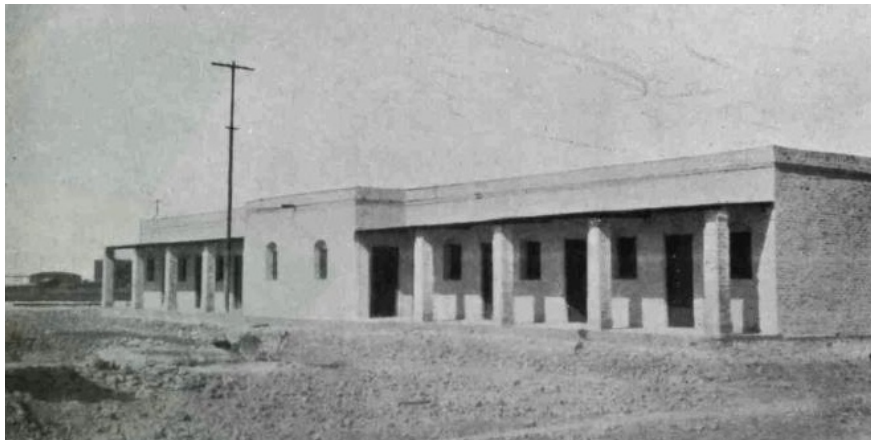
Figure 4.22 New Single Clerks' block under construction, October 1924. Each block consisted of eight rooms and two dining rooms, accommodating 8 men. Each room featured two windows and one door opening onto a verandah.
