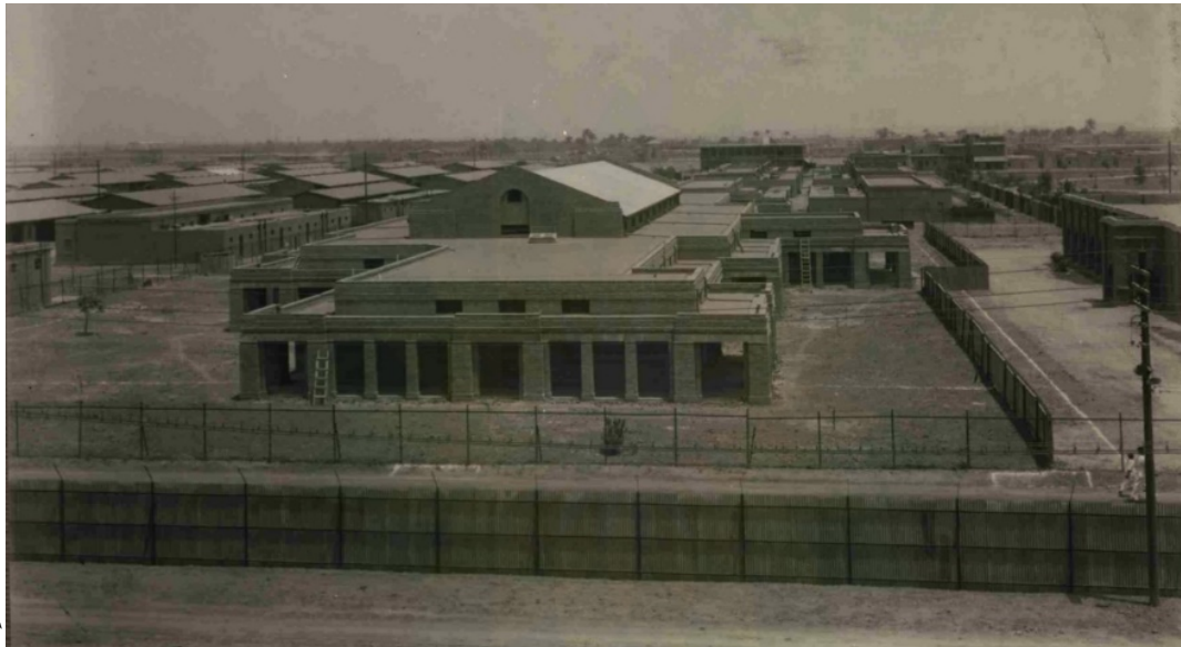
Figure 4.13 A view of the Abadan Out-patient Department from the Refinery looking east, June 1932. Inspired by the environmental control strategies employed in colonial buildings in India, Wilson used varied elevations for different spaces to facilitate ventilation through clerestory windows and protect the interior against Abadan's blazing sun.
