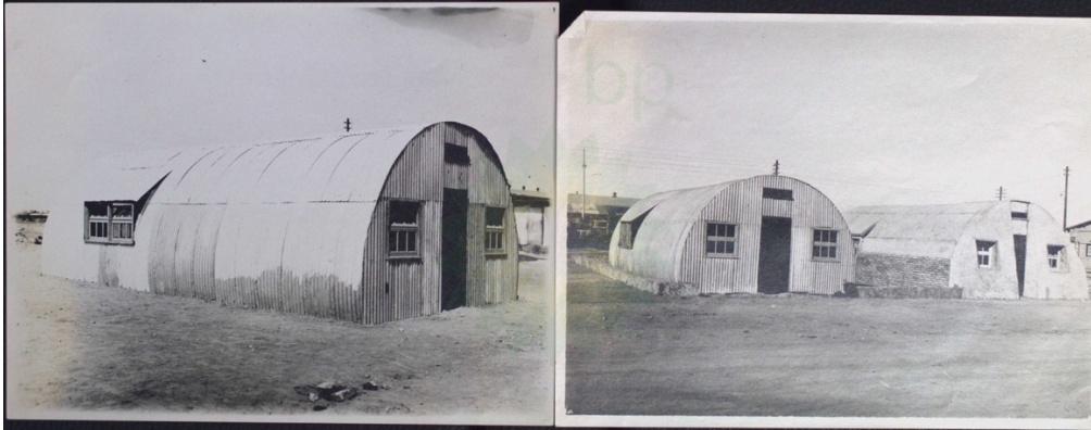
Figure 4.32 Experimental Nissen Huts erected at Abadan, 1930.
