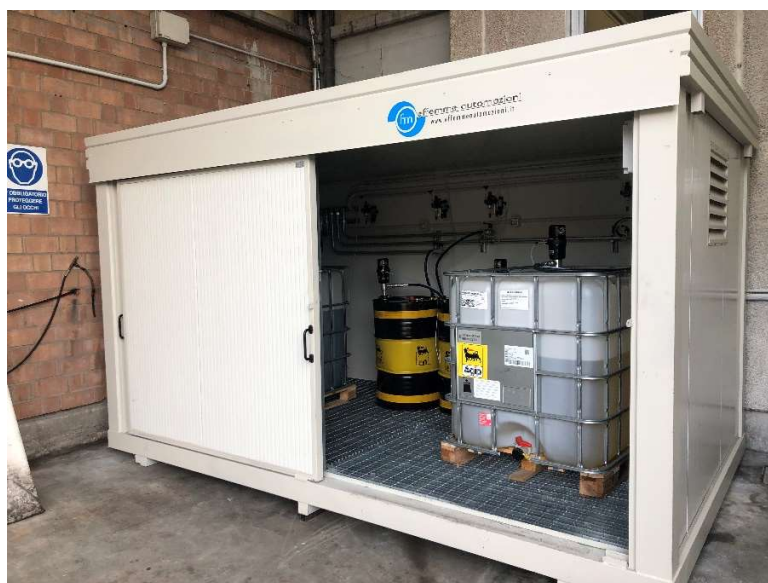
Figure 8.1 The container with the barrels and IBCs of oil.
