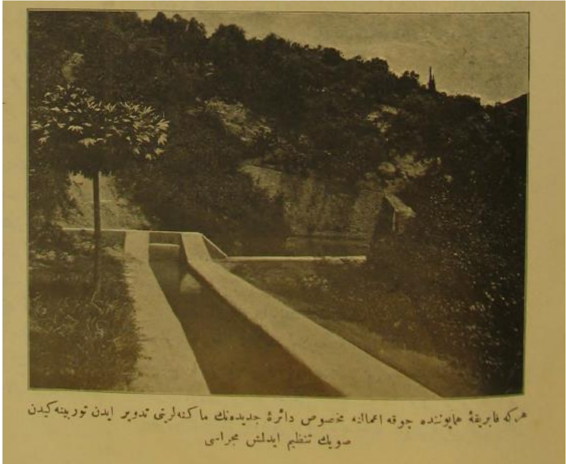
Figure 2.18 The Water Channel.
