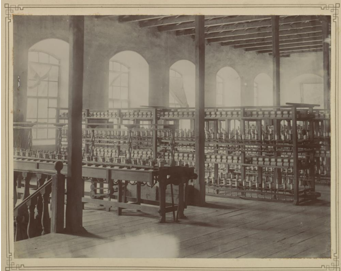
Figure 2.9 Interior of the Filature Building. Source: Istanbul University Rare Works Collection (90453---0024)
