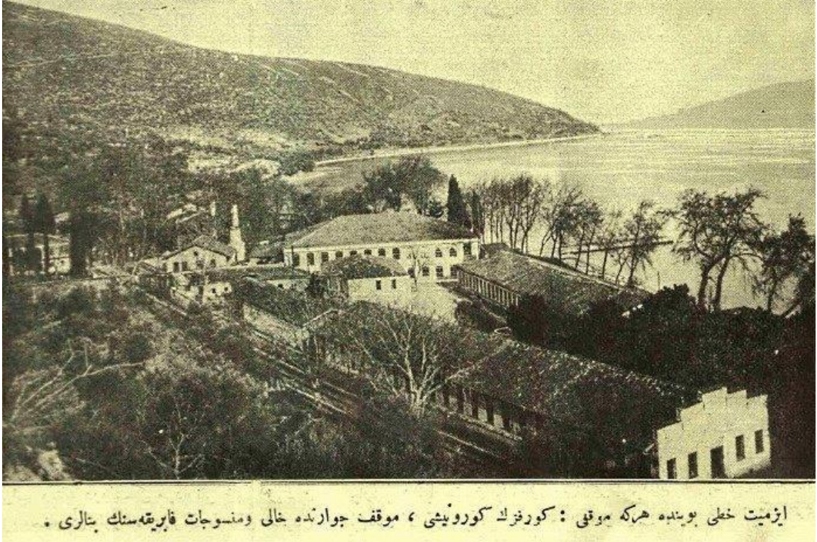
Figure 2.12 Textile Factory and one of the Carpet Workshops at Hereke Factory Campus, ca.1910.
