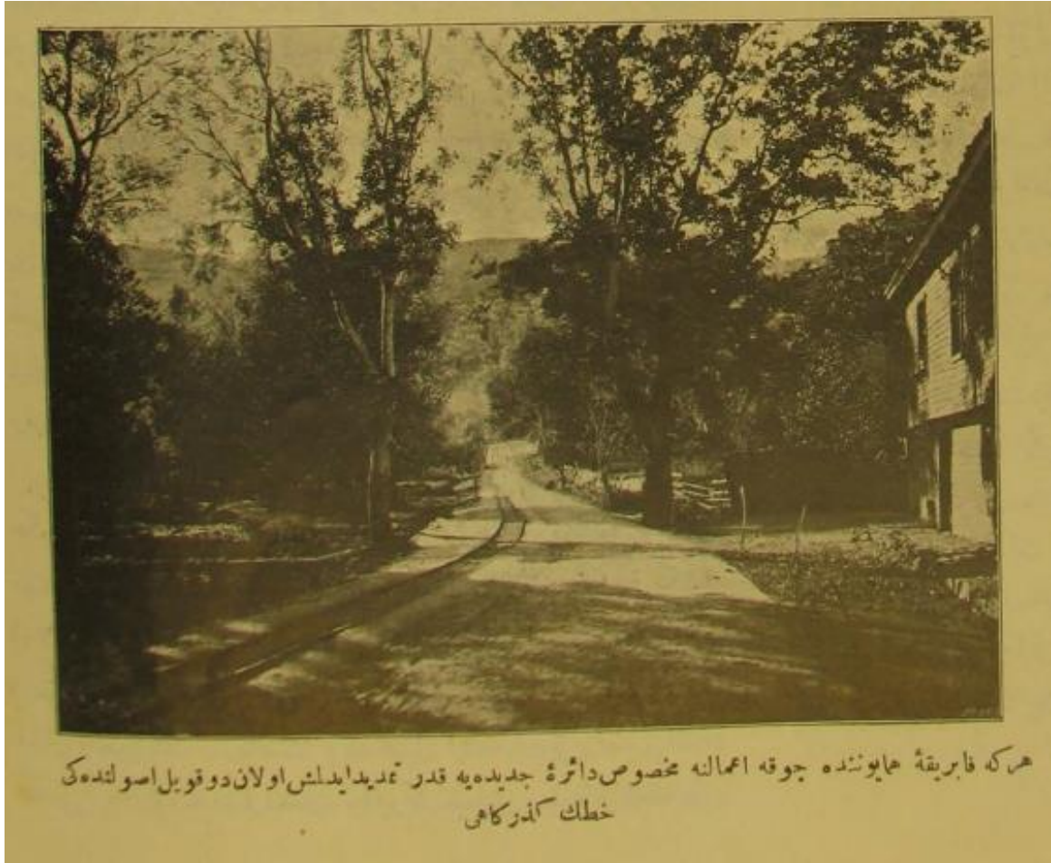
Figure 2.20 The Light Rail.
