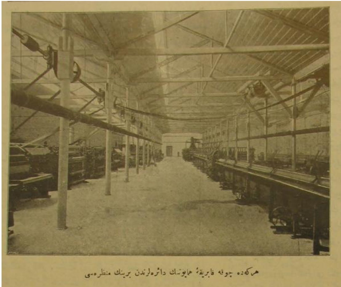
Figure 2.17 Cast iron pillars in the Broadcloth Factory.
