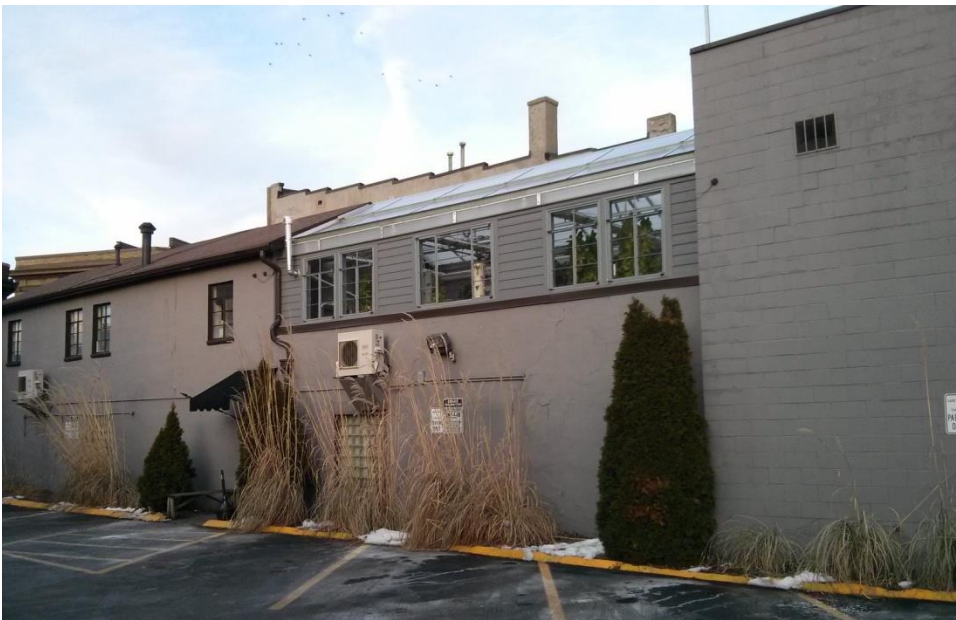
Figure 10.3 Lucky's Taproom's custom greenhouse roof.
