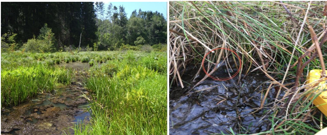
Figure 3.2 Standing water and seepage outflow downstream of the parapet jersey barriers.
