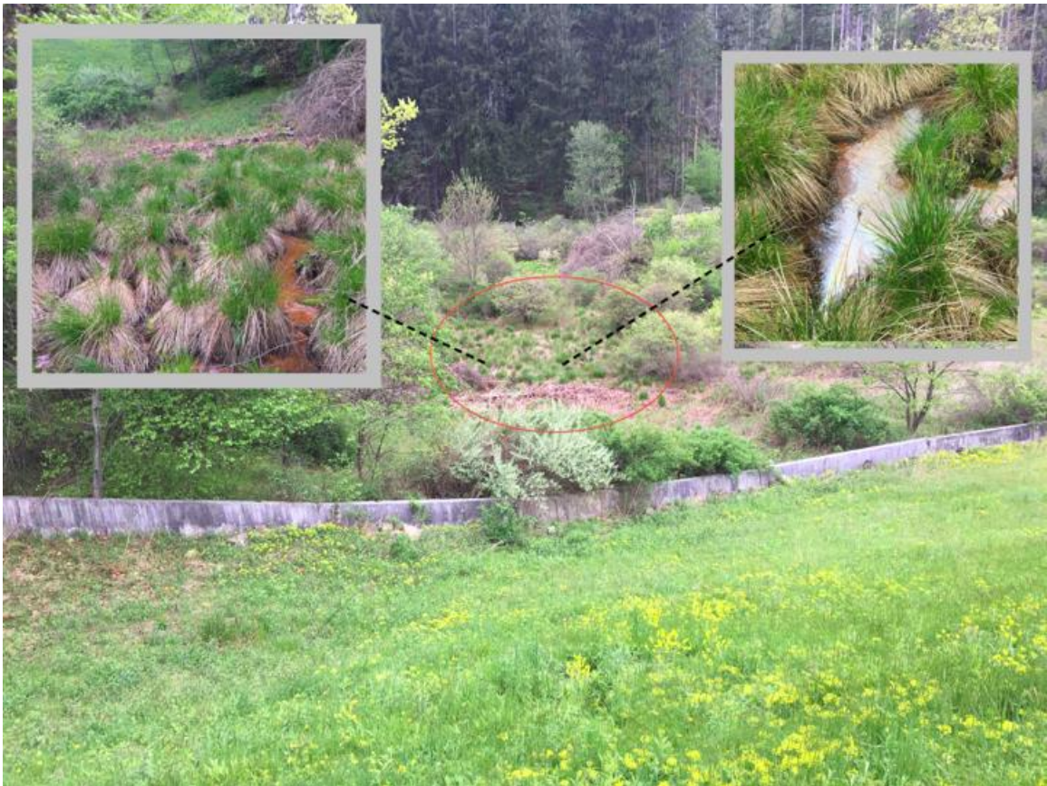
Figure 3.8 Location of standing water downstream of the jersey barriers at station around 2+60.
