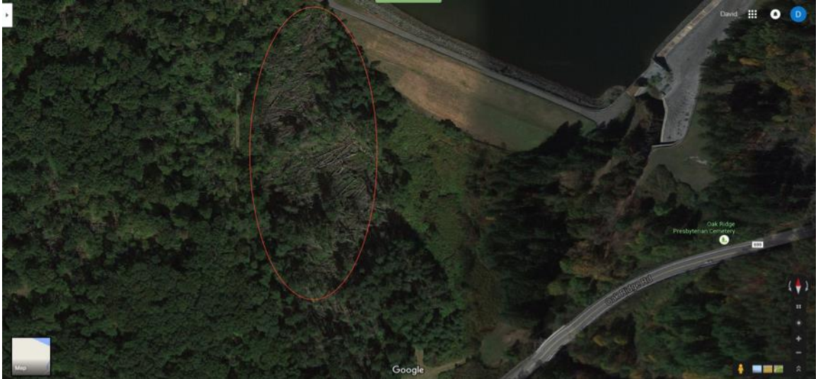
Figure 3.3 Area with the fallen trees downstream of the right abutment
