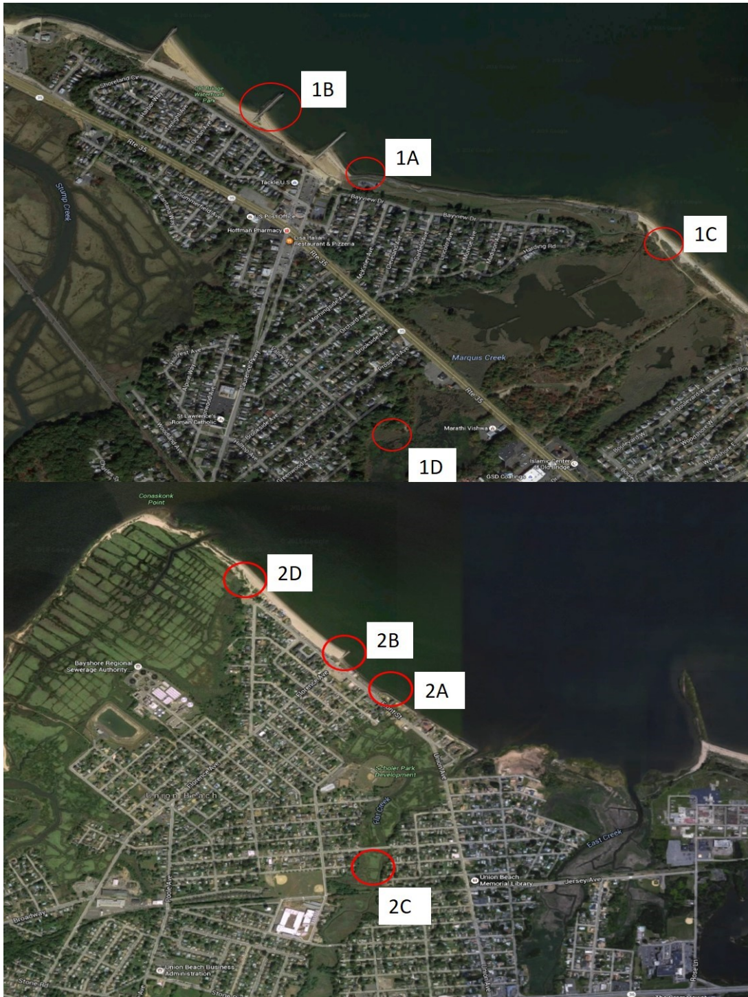
Figure 4.2 Location of engineered structures and natural features (shown in Figure 4.1) from two study areas, Laurence Harbor (1) and Union Beach (2). Laurence Harbor: 1A: Stone revetment; 1B: Groin; 1C: Dune area; 1D: Wetland; and Union Beach: 2A: Retevment and bulkhead; 2B: Groin; 2C: Wetland; 2D: Maritime forest/ dune area.
