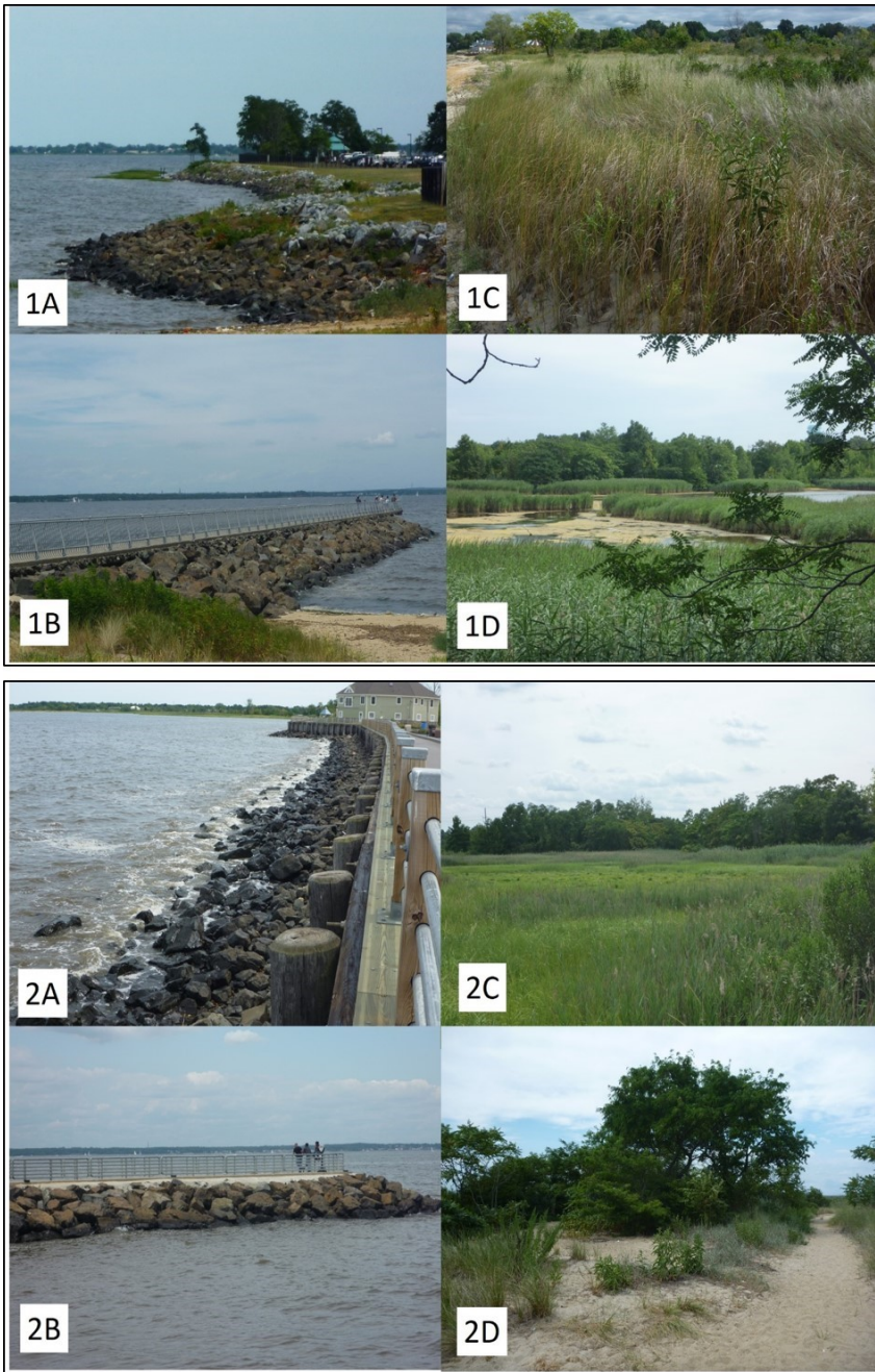
Figure 4.1 Photographs of engineered structures and natural features from Laurence Harbor (1) and Union Beach (2). Laurence Harbor: 1A: Stone revetment; 1B: Second groin; 1C: Dune area on beach near Marquis Creek; 1D: Wetland of Marquis Creek south west of Route 35; and Union Beach: 2A: Revetment and bulkhead; 2B: Groin; 2C: Wetland of Flat Creek; 2D: Maritime forest/ dune areas at Conaskonk Point. Photos A and B represent engineered infrastructure and photos C and D represent natural infrastructure. Source: Taken by researcher on August 8, 2015
