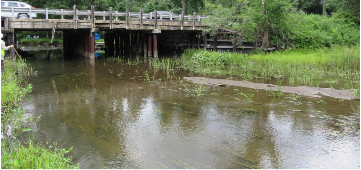
Figure 2.4 Contraction scour, bridge # 1404-158.
