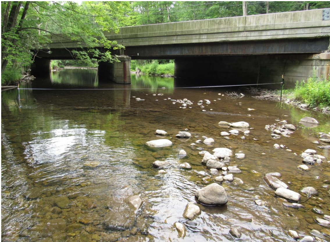
Figure E.28 Bridge # 1912-160 elevation, up-stream looking down-stream, and Wolman Pebble Count section installation.
