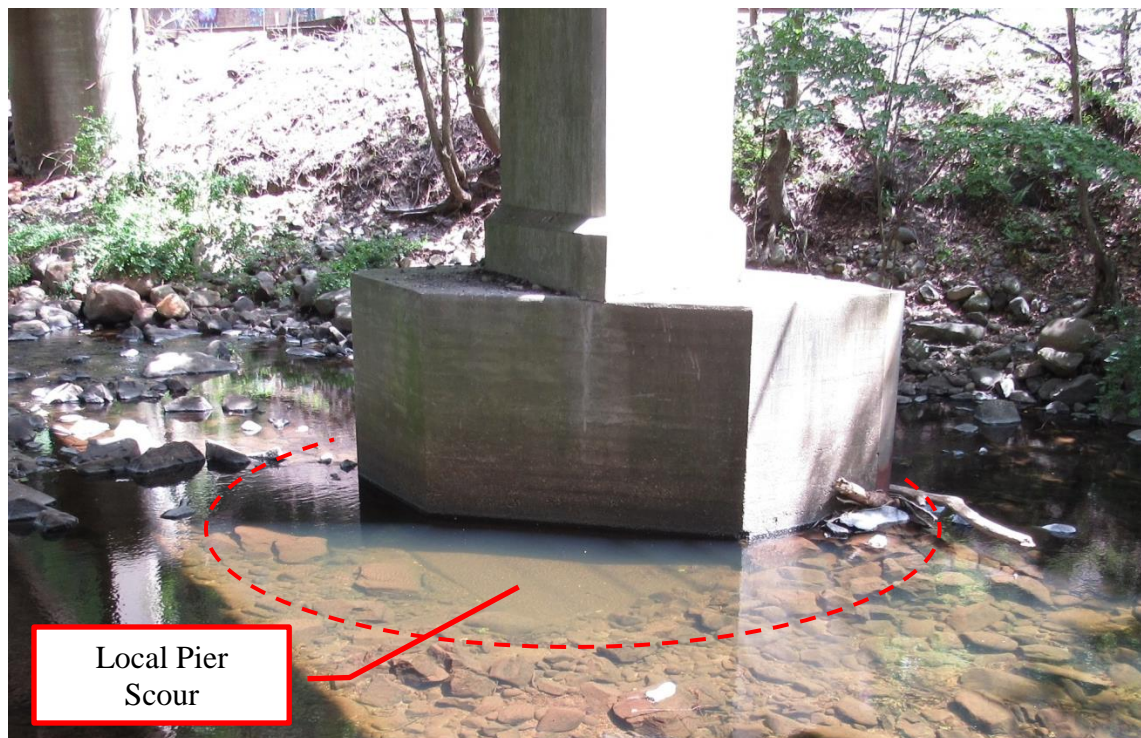
Figure 2.7 Local scour at a pier, bridge # 1405-156.
