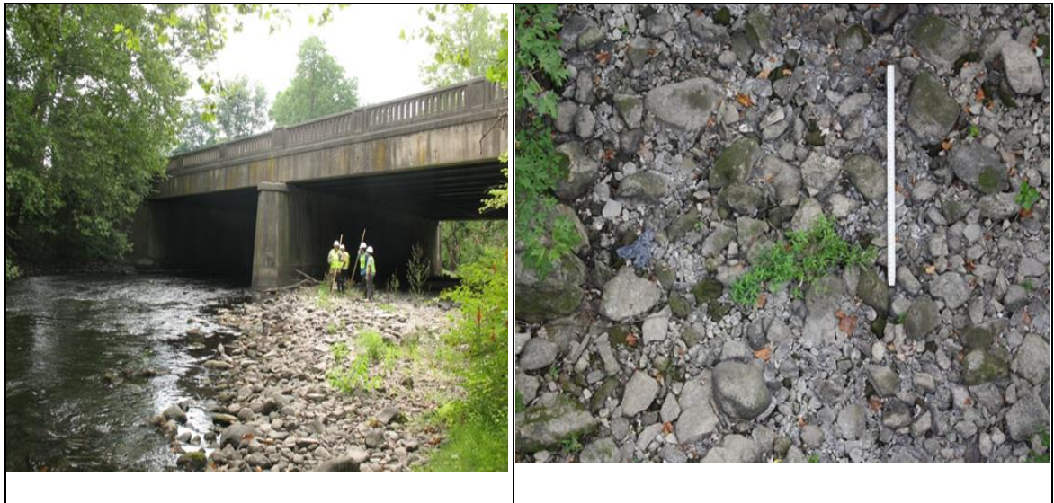
Figure F.1 Elevation and a sample of streambed sediments, bridge # 2107-156.
