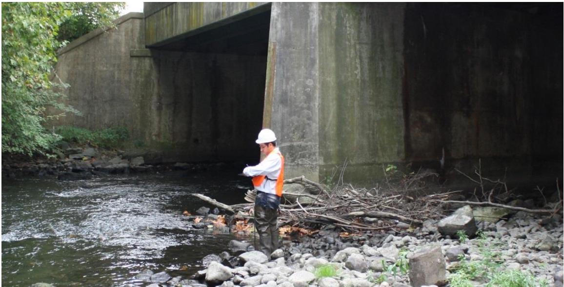
Figure 2.5 Debris build-up in the waterway, bridge # 2107-156.
