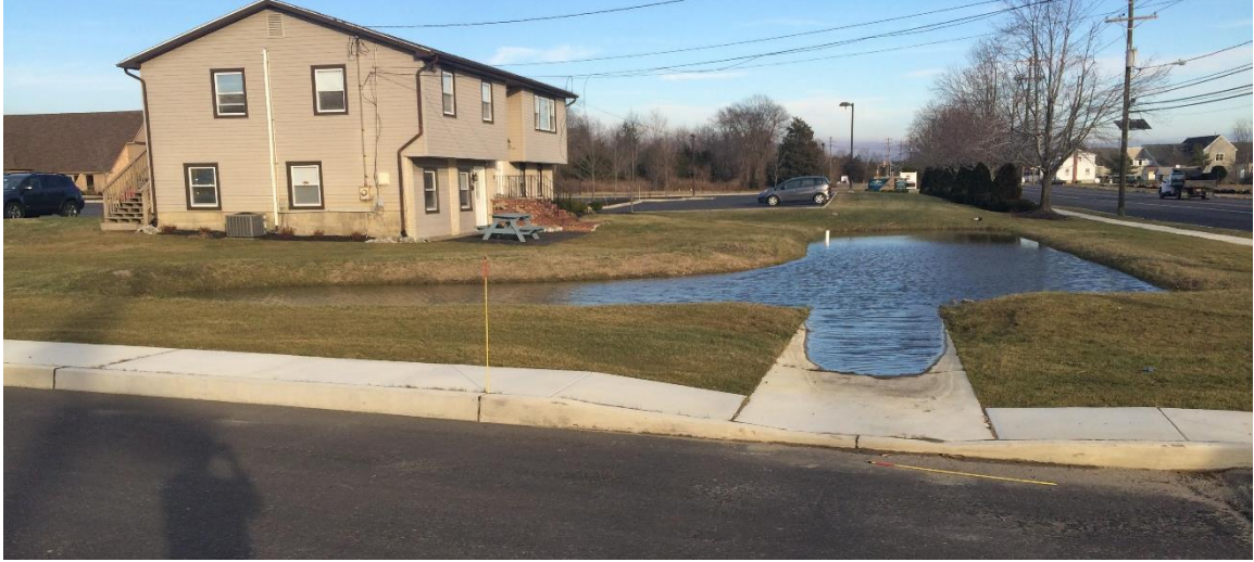
Figure 2.4 Photograph of site detailing inlet.
