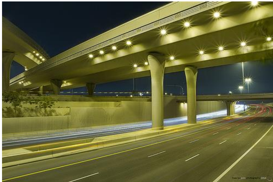
Figure 2.63 Side view of the bridge.
