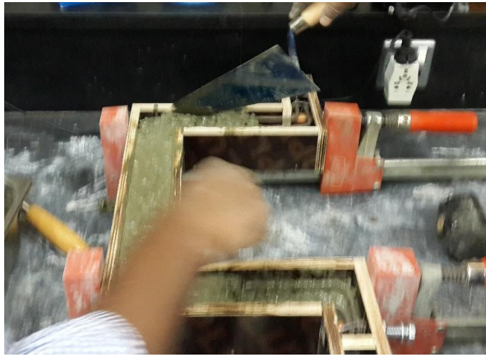
Figure A.4 Pouring the concrete.
