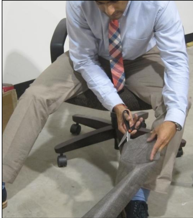
Figure A.3.28 Cutting of Geotextile Fabric Filter Layer
