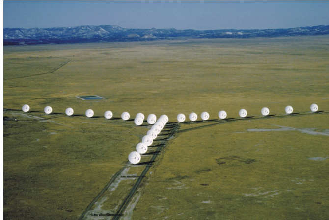
Figure 3.1 VLA array in Y shape configuration.
