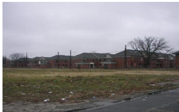
Figure 5.20 Vacated buildings at Roosevelt Manor waiting demolition.
