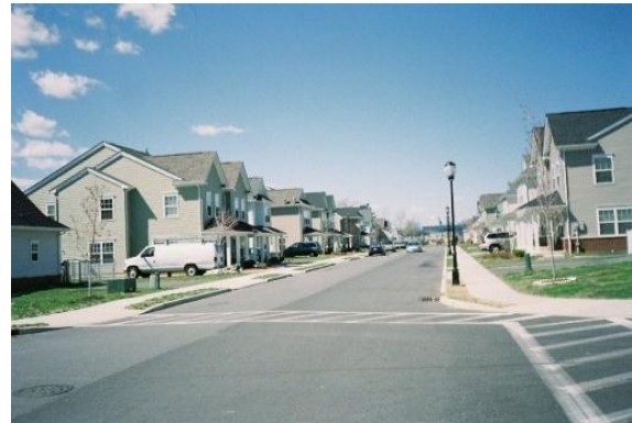
Figure 5.15 Baldwin's Run two-story units on N 31 st St. Shows some of the two-story units with pitched roofs, front porches, and off-street parking.
