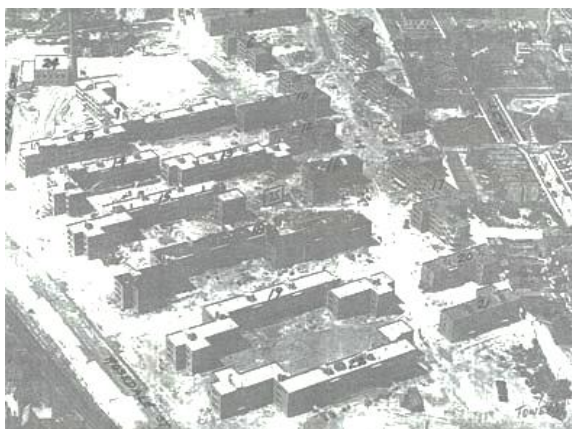
Figure 5.10 Aerial view of Westfield Acres buildings and layout before demolition.
