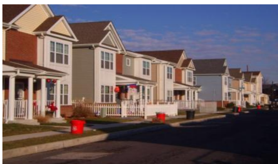
Figure 5.23 Town-house Units at Roosevelt Manor.
