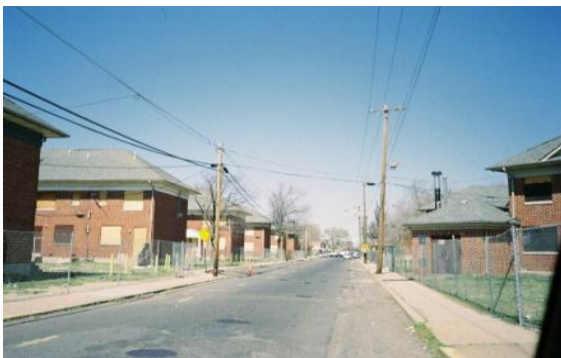
Figure 5.19 Vacant Roosevelt Manor Buildings Awaiting Demolition, Spring 2007.
