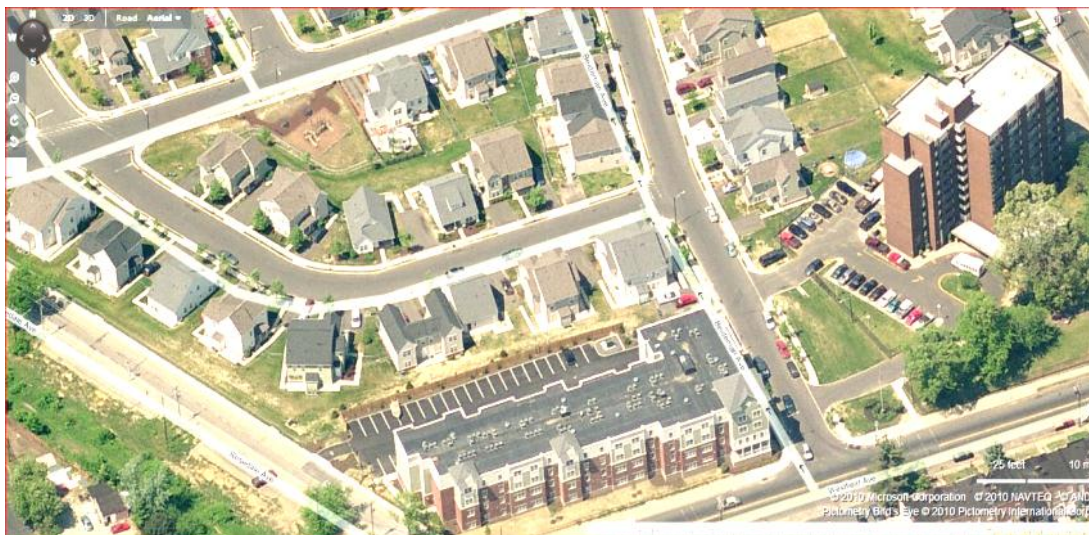
Figure 5.12 Aerial View of Baldwin's Run showing public housing units on Baldwin's Run Lane on left side. The four-story building at the bottom of the picture is Baldwin's Run Seniors building. The right side of picture shows Westfield Towers (for seniors).
