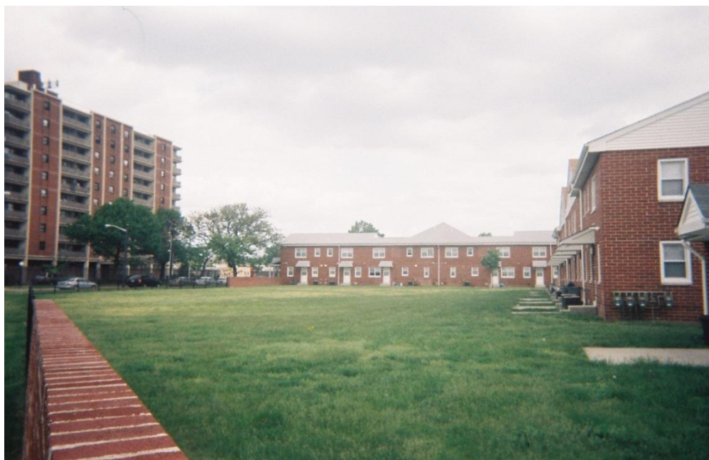
Figure 5.4 A shared backyard surrounded by a perimeter wall along Watson Street near the HACC Head office and two rows of residences. Shared backyards typically look like this one. Kennedy Towers, which house elderly residents and the HACC administrative offices, is the high rise building on the left side.
