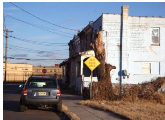
Figure 5.2 Carman Street housing adjacent to McGuire Gardens.
