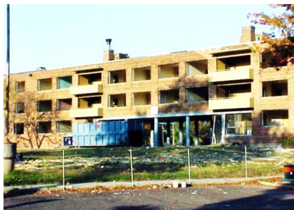
Figure 5.11 A Vacant Apartment Block at Westfield Acres Before Demolition in 2001.
