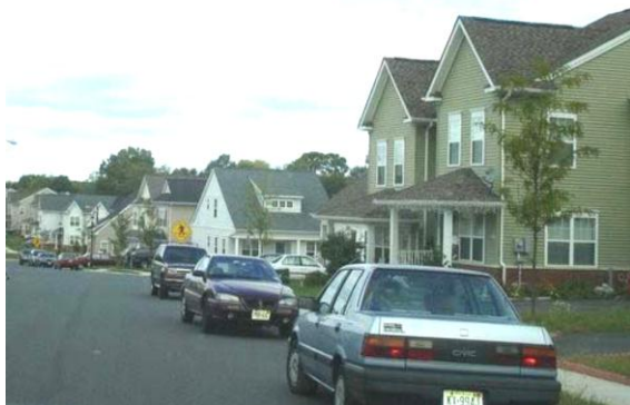
Figure 5.16 Baldwin's Run Twin Units on 32 nd Street. Twin style housing is in the foreground and detached single-family units are further down the street.
