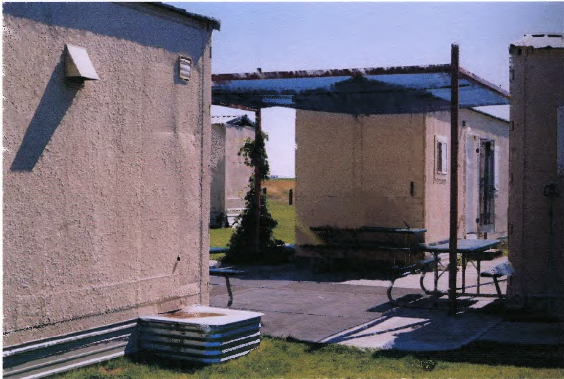
Figure 3.4 Covered outdoor court shared by four units. (Source: Palleroni)
