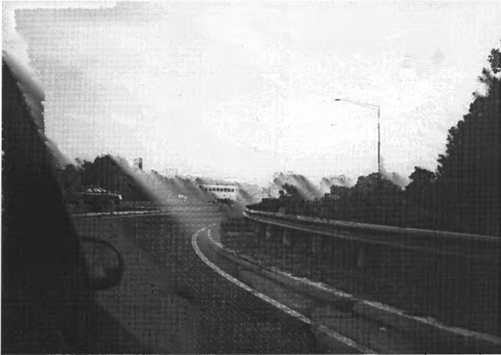
Figure A.5 Ramp 1 on I-80 (Route 615/Howard Boulevard).
