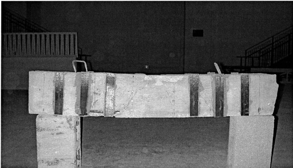
Figure 2.13 Failure of Beam Z4-90.
