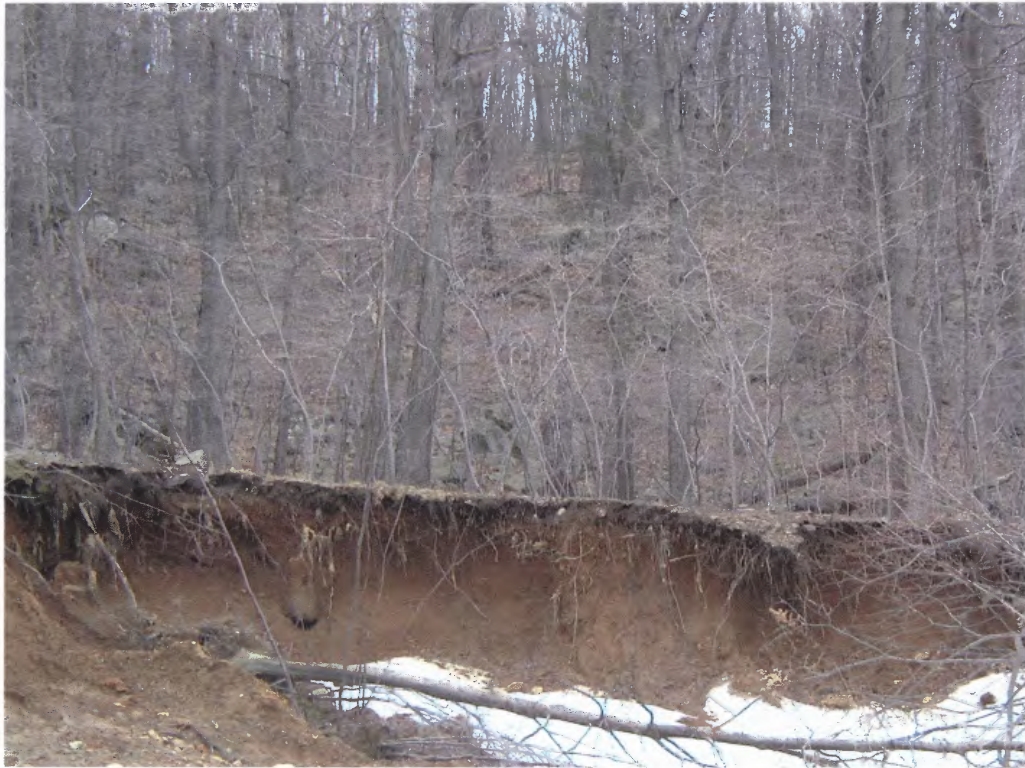
Figure 3.8 Photograph of left flank of landslide.
