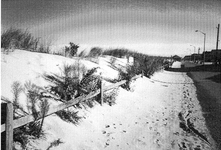
Figure 10 Photograph, looking south, showing landward side of dune and boardwalk at Site 8 in Manasquan, NJ.
