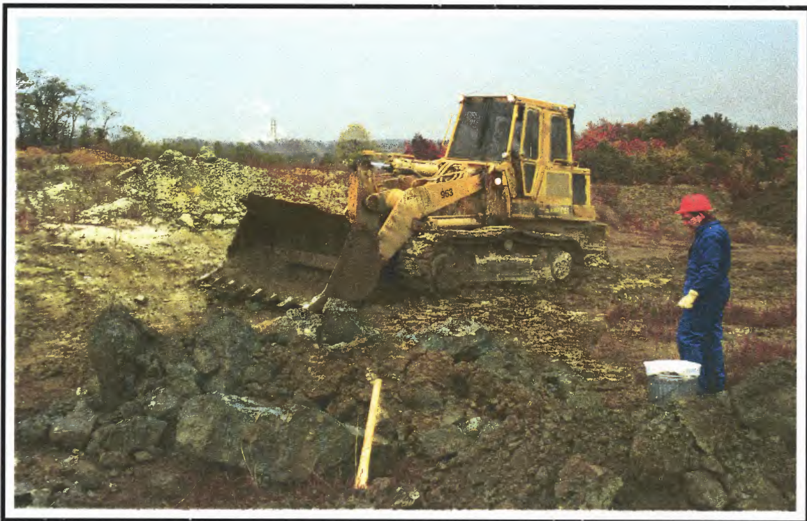
Photograph A-3. The Potomac Formation clays required excavation by a bulldozer. The blue and red clays are shown to the left and right, respectively.
