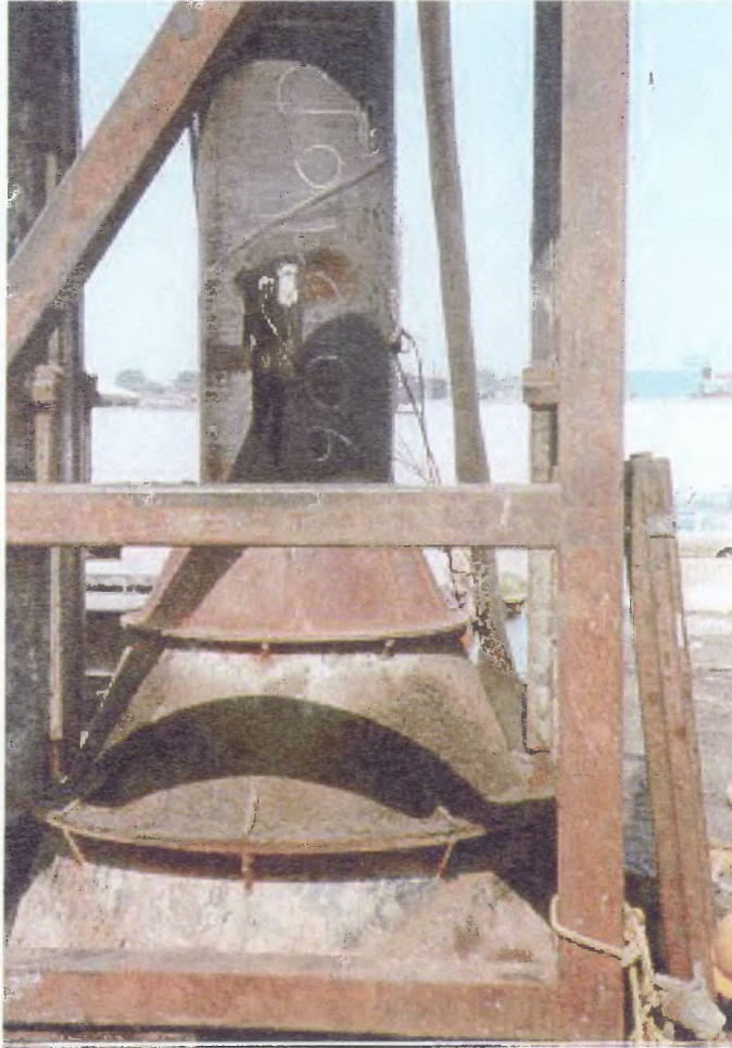
FIGURE 3.3 Strain Gauge and Acceleration Transducers Connected to Pile for Dynamic Load Test
