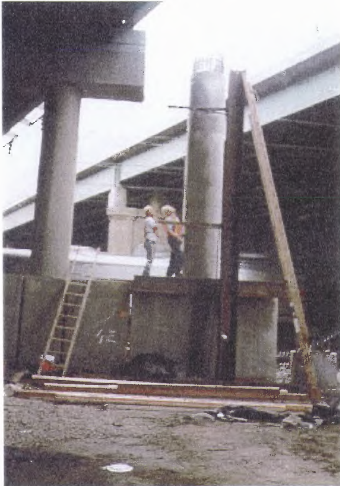
FIGURE B.10 Pier Construction for I-78 Widening
