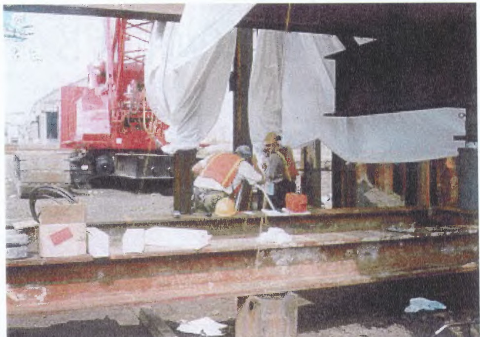
FIGURE B.9 Checking of Uplifting of Reaction Frame
