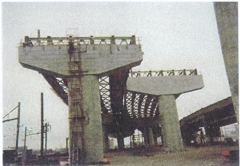
FIGURE B.11 Pier Construction for Route 21 Viaduct
