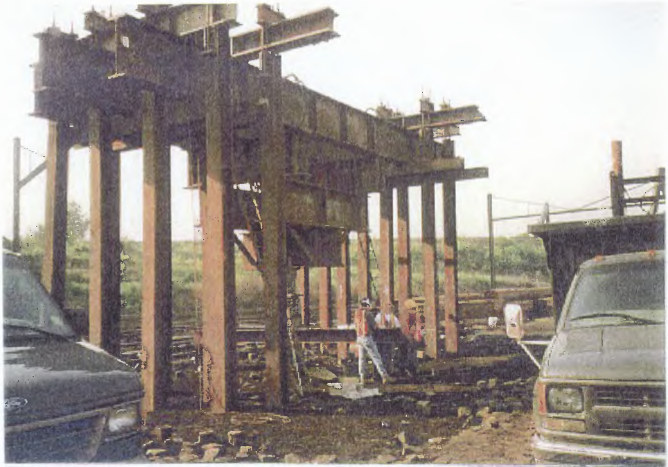
FIGURE 3.5 A View of Static Load Test Reaction Frame
