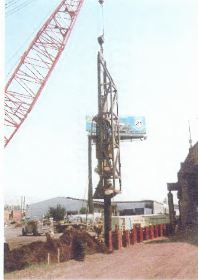
FIGURE 3.4 Dynamic Load Test near Route 21 Rail Lines
