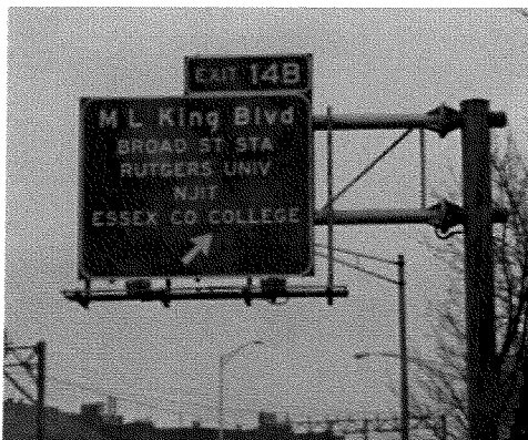
Figure 49. Cantilevered road sign between exits 15 and 14.
