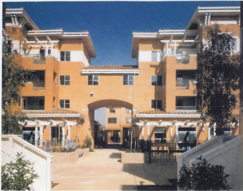
Figure 30: Photograph of Hismen Hin-nu Terrace by Michael Pyatok. (Jones, Pettus, and Pyatok, Good Neighbors: Affordable Family Housing , p.101)
