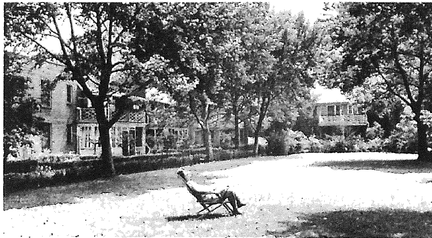
Figure 14: Courtyard at Sunnyside Gardens. (Stein, Toward New Towns for America , p.30)
