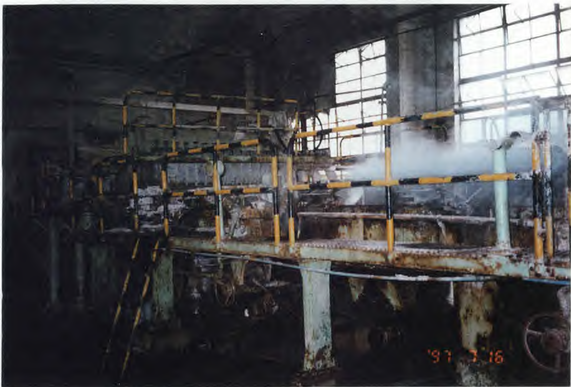
Photograph 11. The Paper Machine with Wire-Mesh Conveyor Belt
