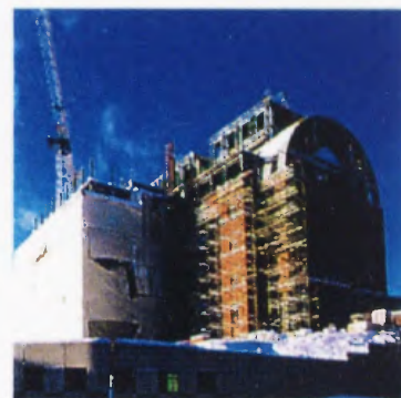
NORTHEAST CORNER: Steel truss vault.
