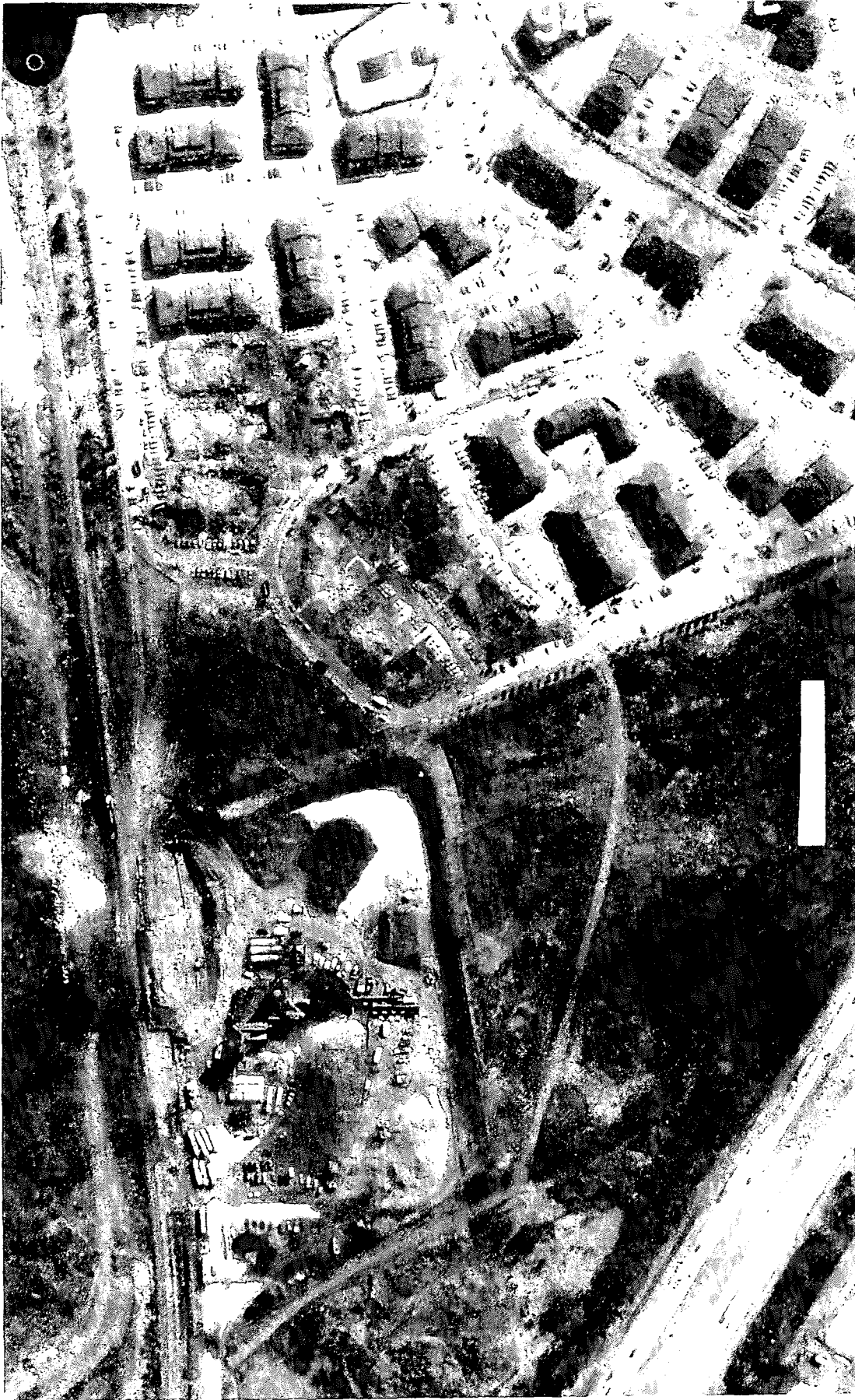
Figure C.1 - Detailed View of Edison Accident
