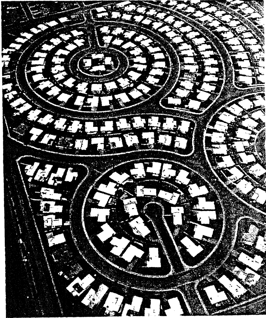
Figure 4. An example of a curved street pattern employed by the developer, differing --and disconnecting-- the development from the surroundings. Note the grid of streets that starts at the top of the development. (Southworth and Ben-Joseph, 1996)
