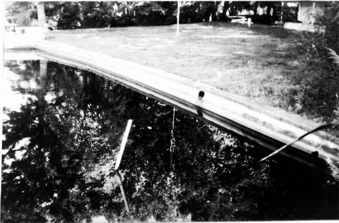
Figure 2d Picture showing "Concrete" reference bulkhead
