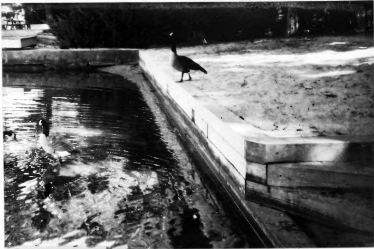
Figure 2c Picture showing "Wood" (CCA) bulkhead.
