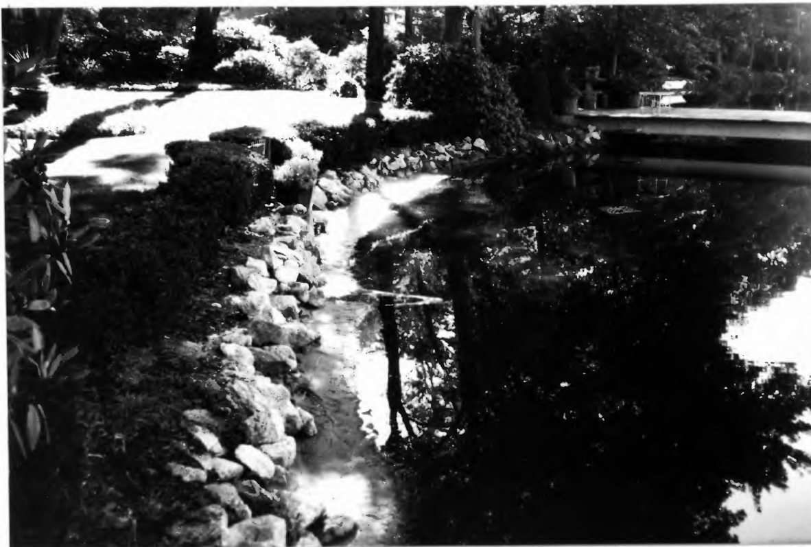
Figure 2b Picture showing "Rock" reference bulkhead
