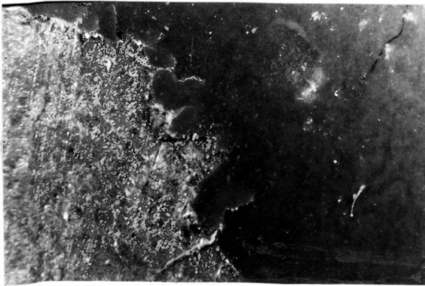
Fig. A.142 Micrograph of cracks, tearing at boundary of oil-based paint and substrate after waterjet coating removal.
