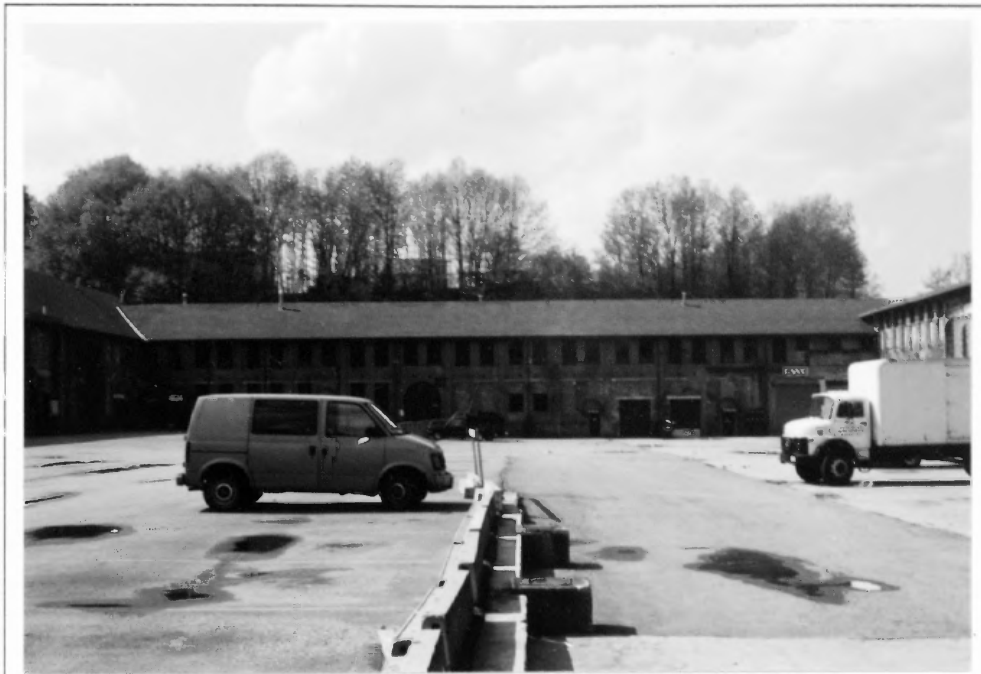
Fig.30. Building #2, south facade
