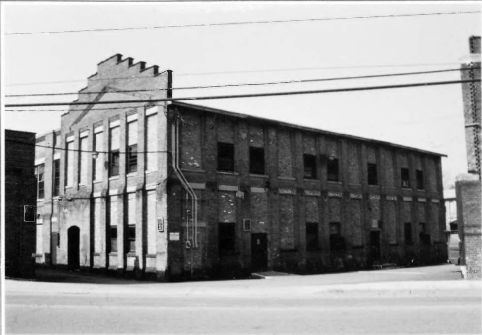
Fig.34. Building #8, south facade
