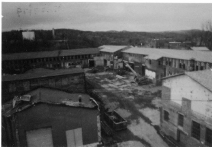
Fig. 53. Butler complex during demolition
