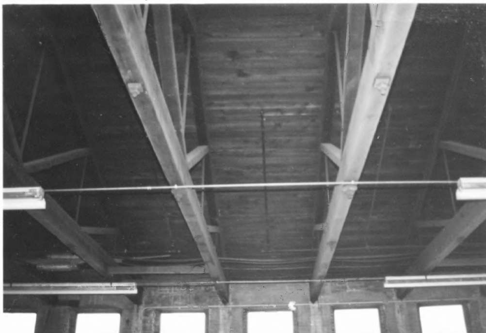
Fig.49. Wood truss roof structure
