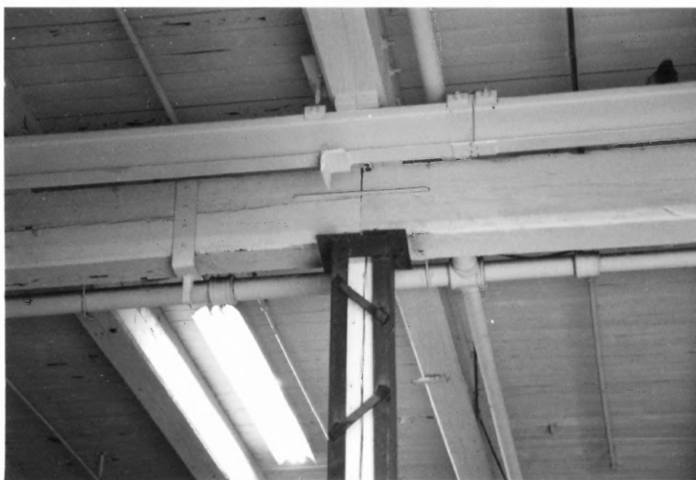
Fig.50. Reinforced heavy timber post and beam structure
