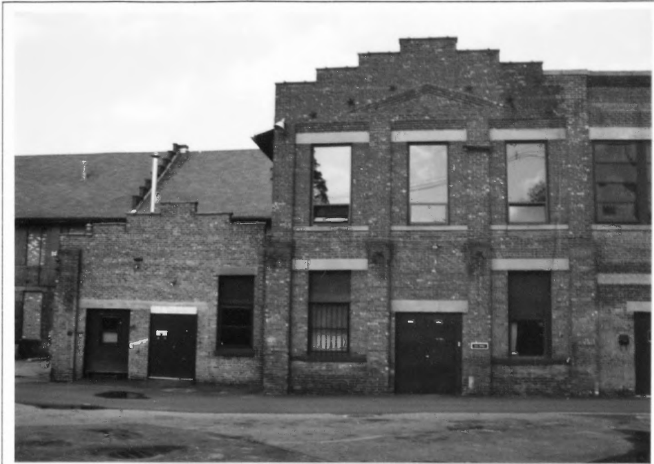
Fig.33. Building #7, west facade
