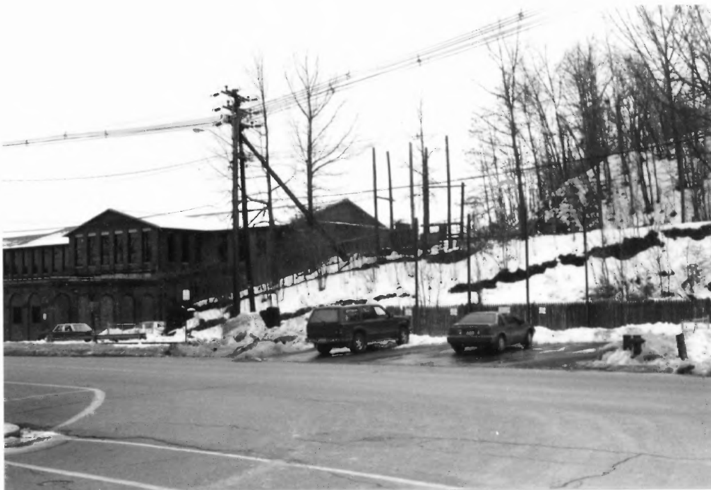
Fig.25. Steep embankment to the north of Butler Center
