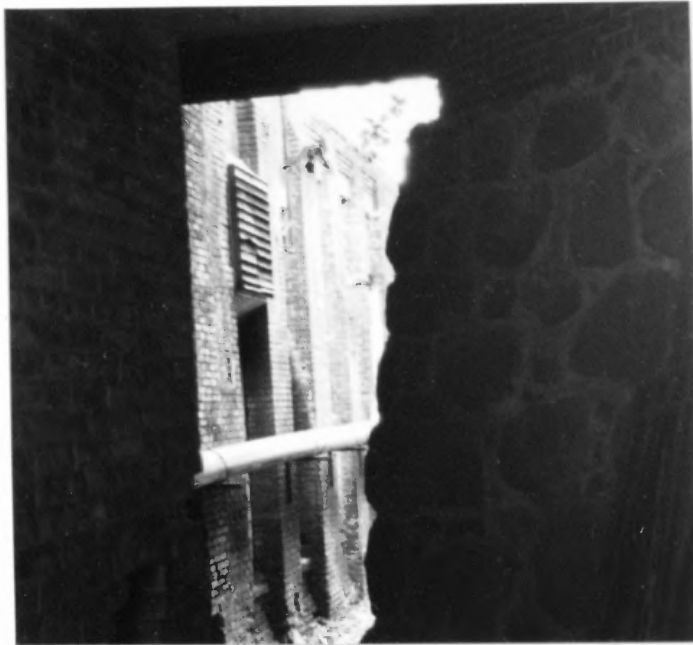
Fig.43. Retaining wall to the north of Butler Center
