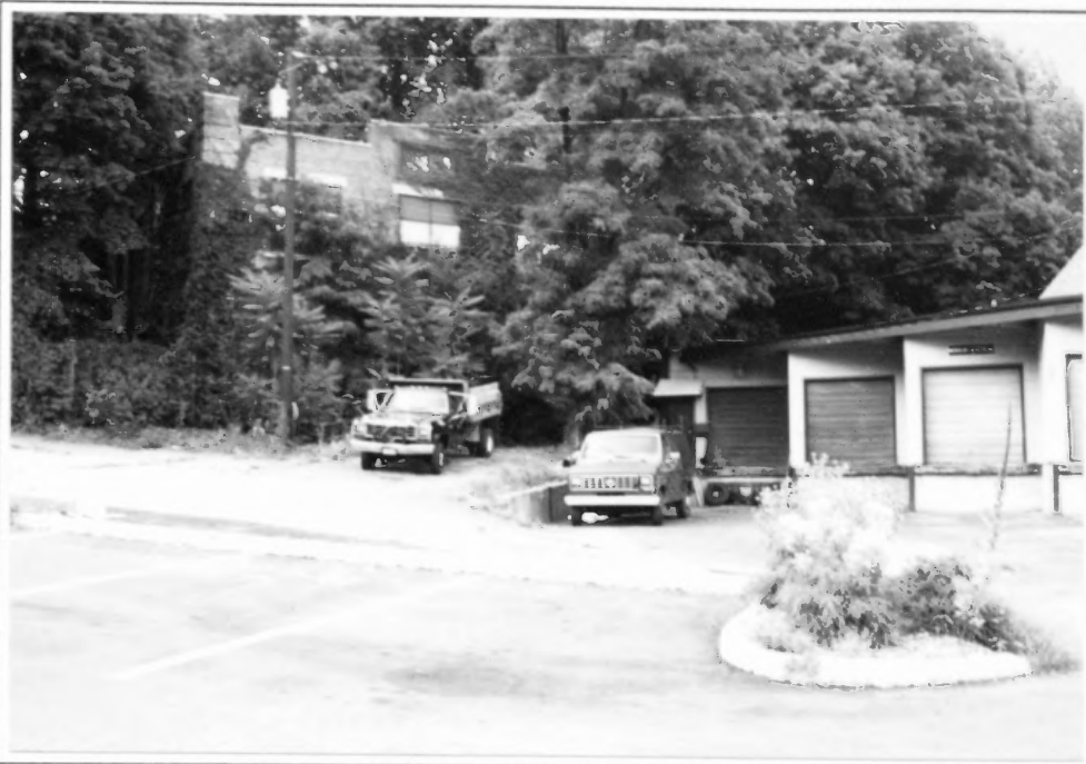
Fig.40. Building #16, south facade
