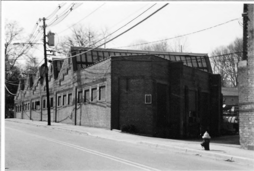
Fig.38. Building #14, south facade
