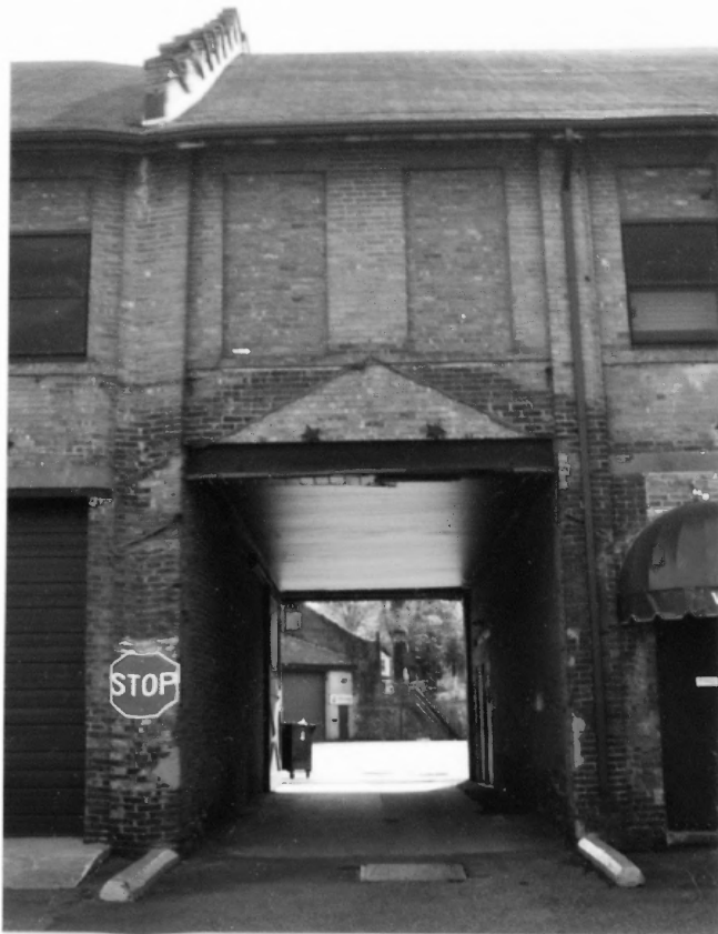
Fig.74. Drive-through of building #3
