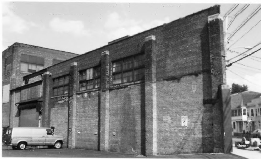
Fig.63. Vehicle bay, west elevation of building #15
