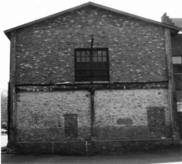
Fig.41. East facade of building #8
