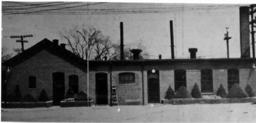
Fig.66. Butler Police building 1950
