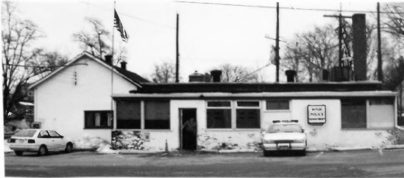
Fig.65. Butler Police building 1995
