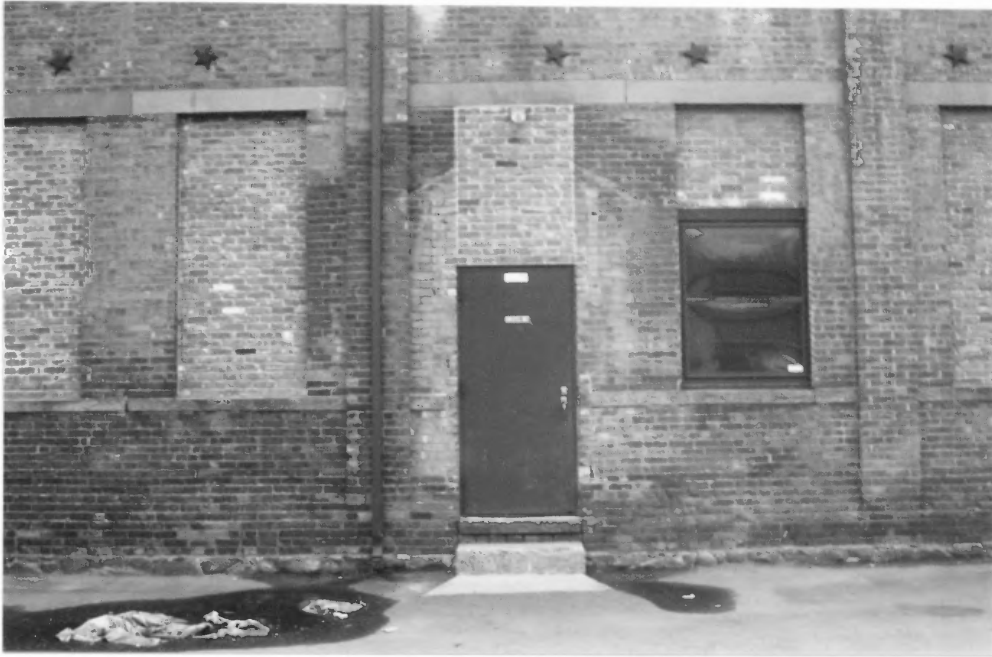
Fig.45. Infilled windows, east facade building #3
