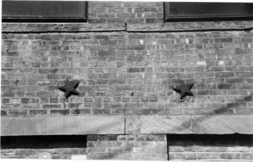
Fig.47. Star-motif tie rods and dressed sills and lintels
