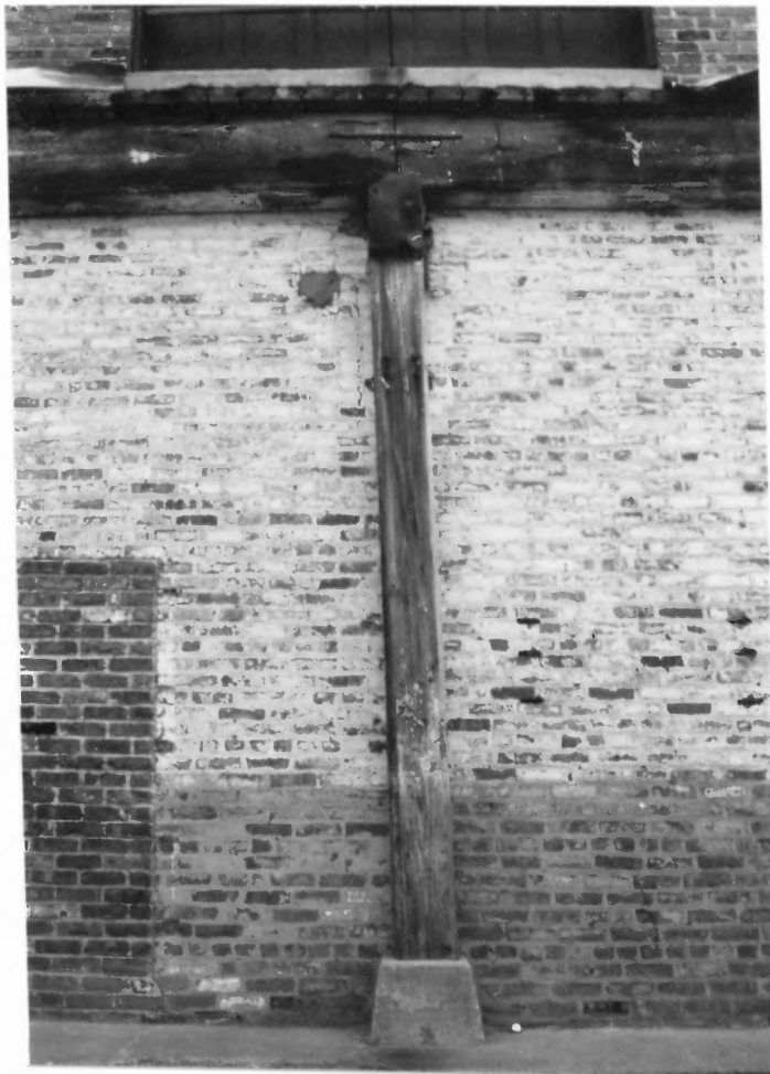
Fig.44. Exposed structure of building #8
