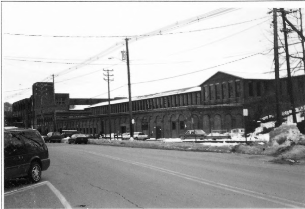
Fig.37. Building #13, east facade
