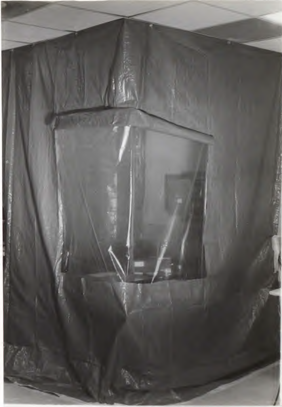
Figure 6a Canvas enclosure for vibratory equipment.
