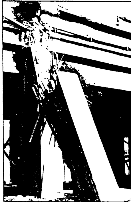
Figure 1.11 Failure of the West Side of Bent 90
