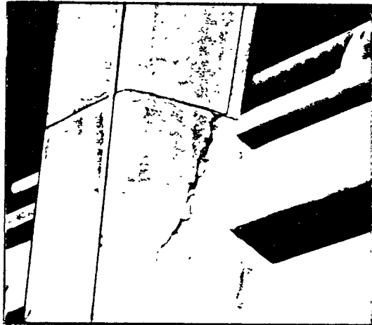
Figure 1.8 Cracking Below the West Shear Key, Bent 55
