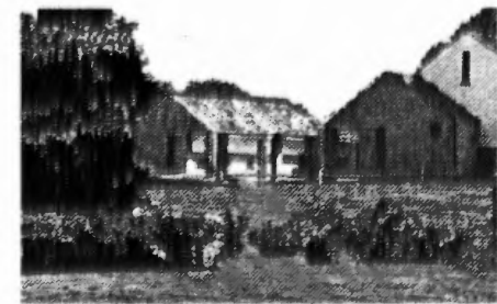
Figure 147. The organic architecture of the structures is reinforced by the romantic development of their gardens.
