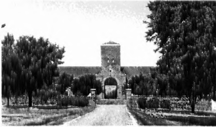
Figure 134. The symmetrical exterior space of the courtyard with its ordered vegetation reinforces the axial, classical style of the house.
