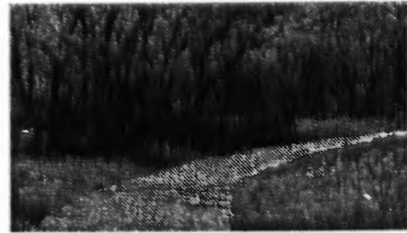
Figure 116. A deflected vista is developed as the road moves past a clump of trees.
