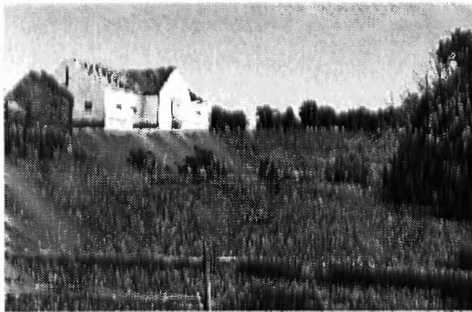
Figure 127. The volume of a house placed at the end of a hedge row balances a clump of trees in the contiguous field.
