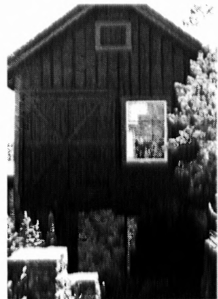
Figure 51. The continuous color of the barn door and the siding create a unified façade, while the different colors of the trim around the window and the upper vent make these elements more visible.
