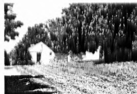
Figure 124. A house is nestled into the existing trees.
