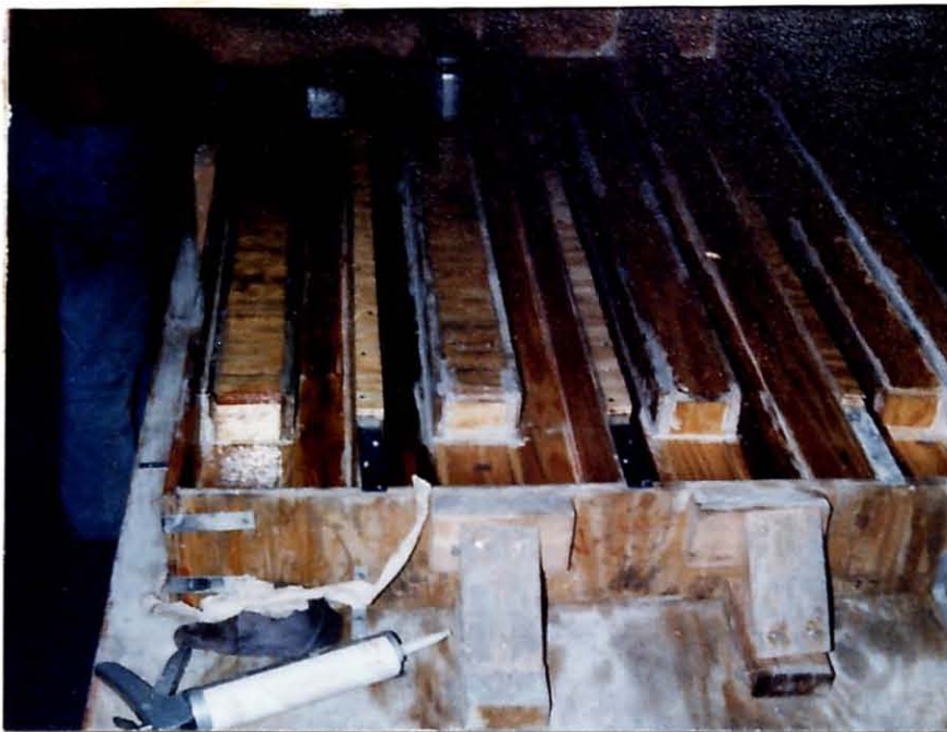
FIGURE 2.3a FORMWORK DETAILS - SHOWING THEM UNFILLED
