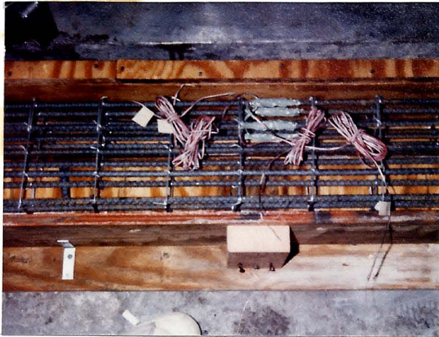
FIGURE 2.6.a STRAIN GAUGE INSTALLATION
