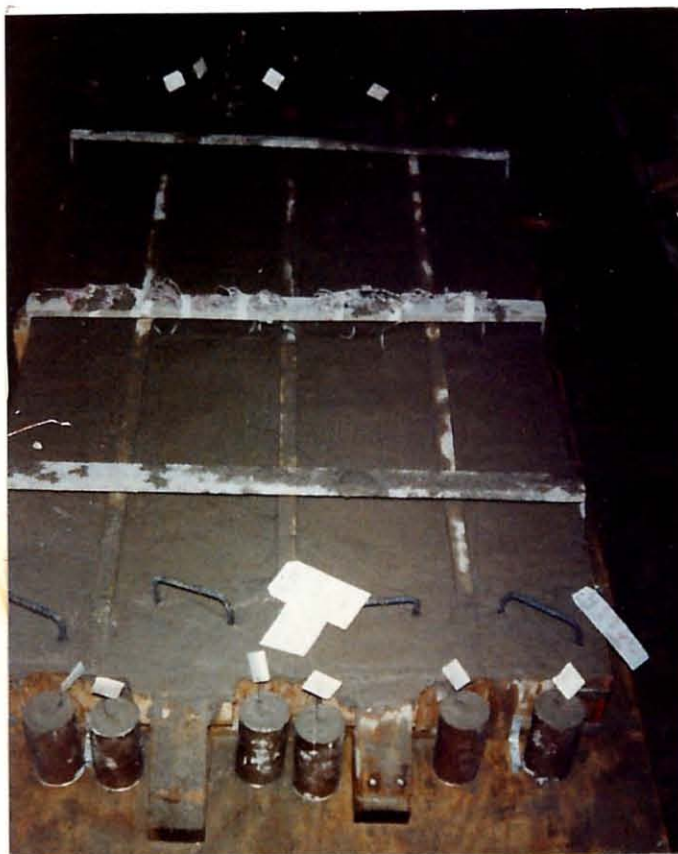
FIGURE 2.3a FORMWORK DETAILS - SHOWING THEM UNFILLED
