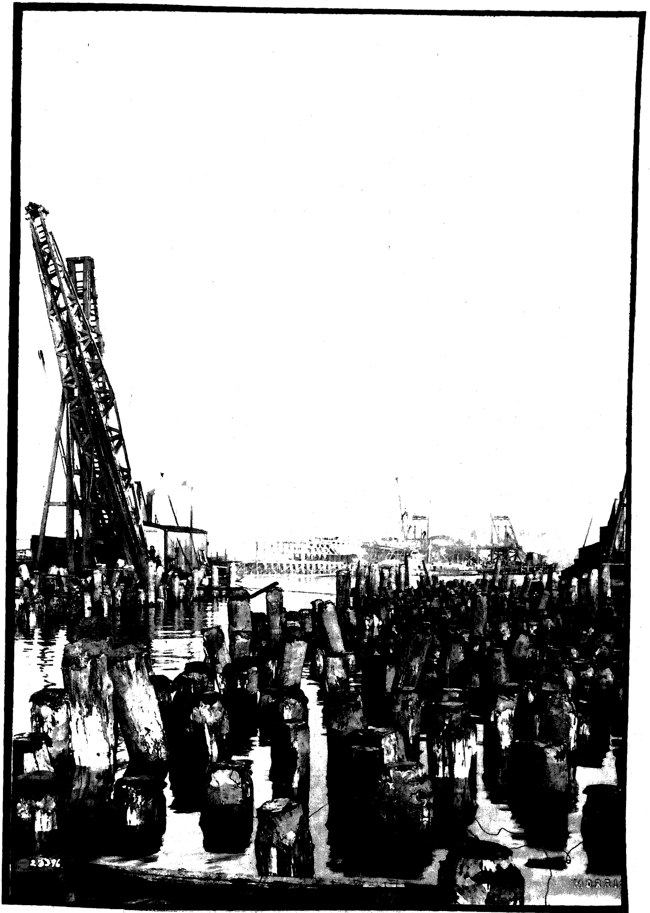
Fig. 71.- Piledriver with pendulum leads.
