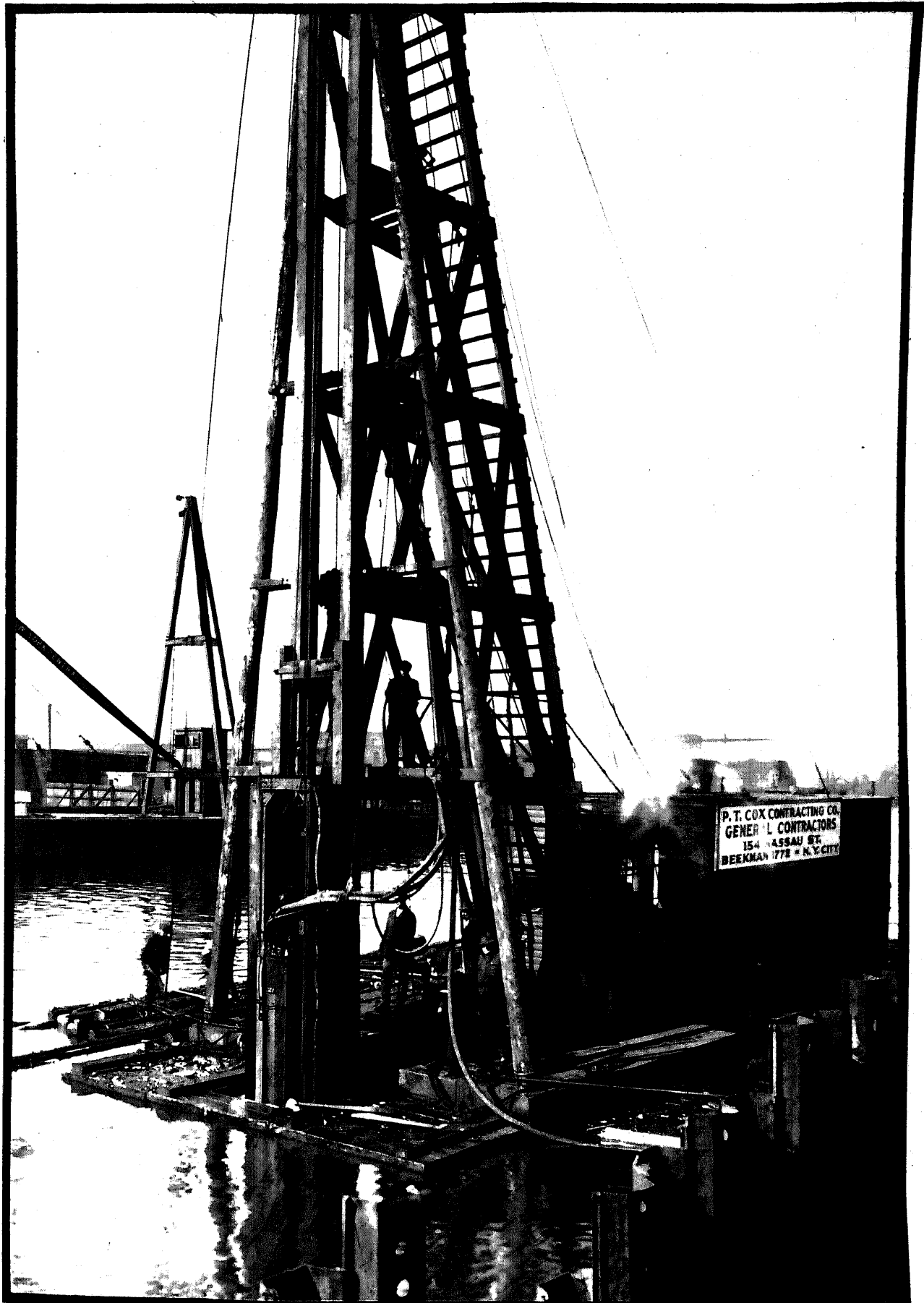
Fig. 70.- Piledriver with telescopic leads.
