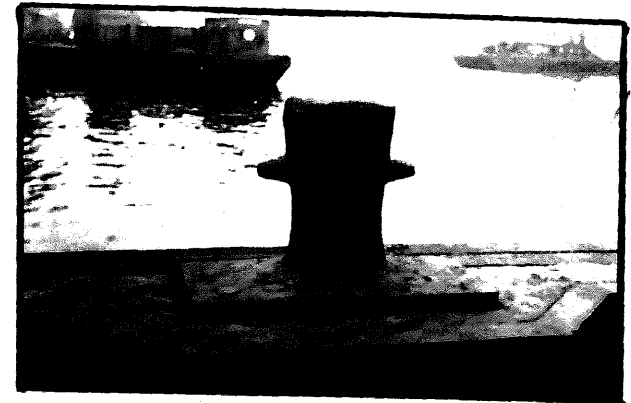
(f) Cast steel single bitt.
