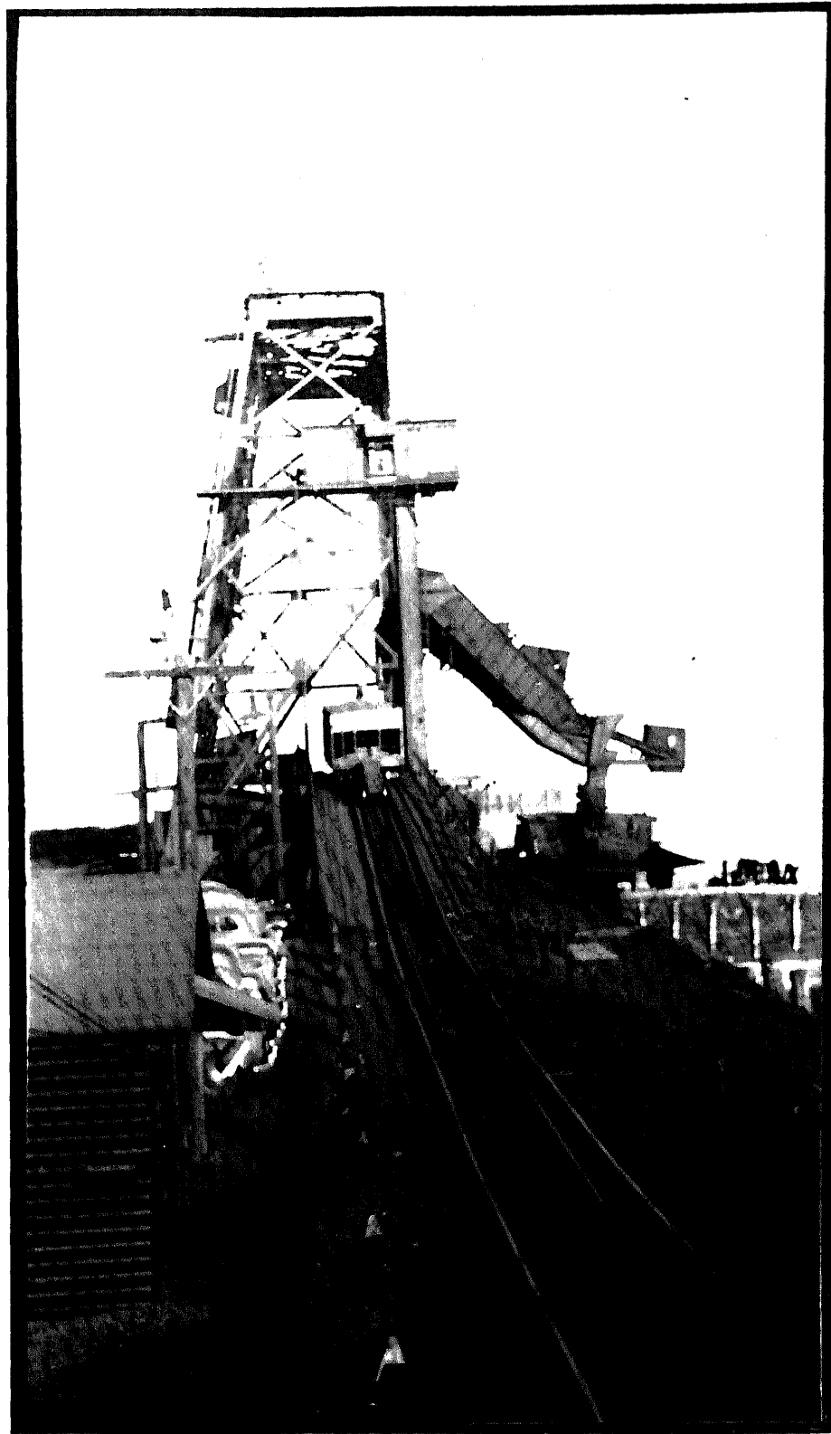
Fig. 21.- Car dumper, Seaboard Coal Dock, South Amboy.
