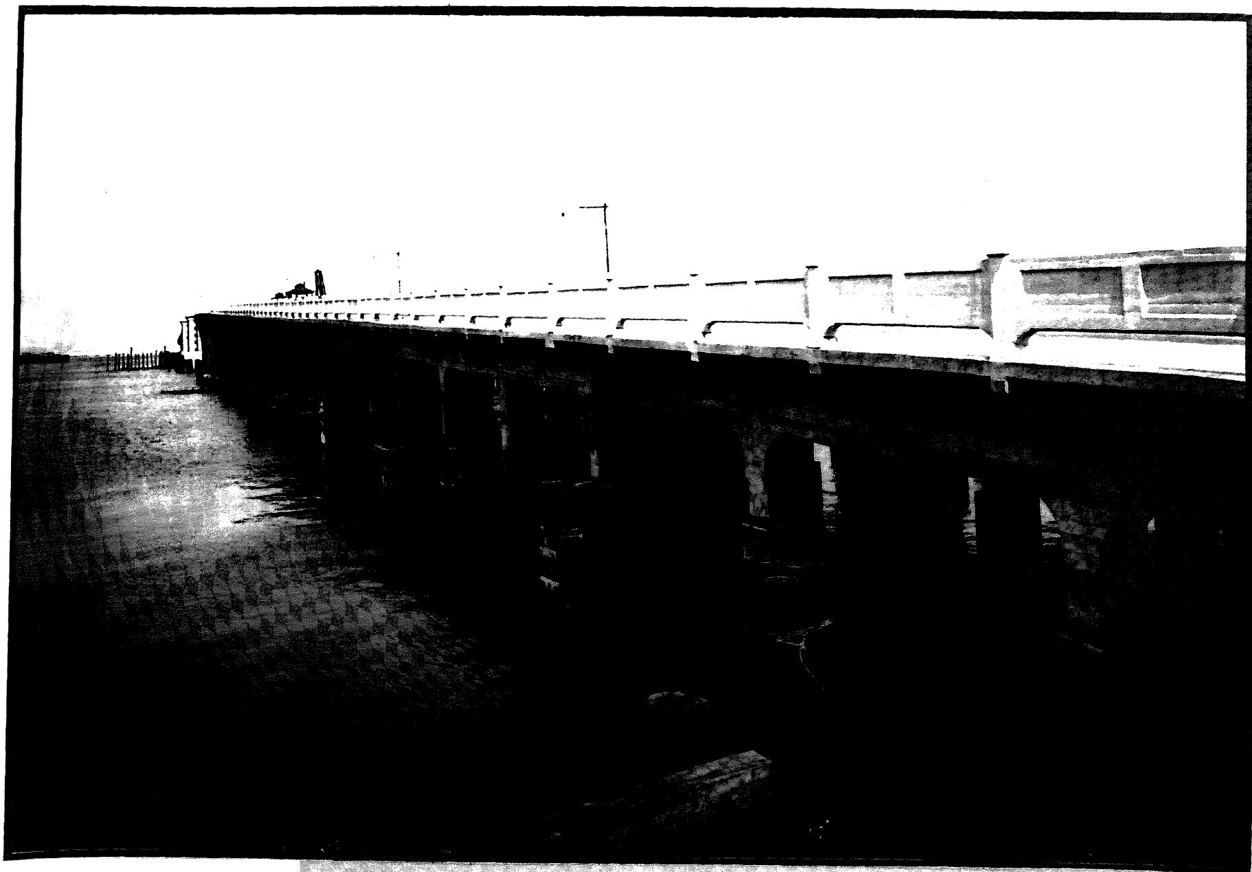
Fig. 31.- Cross-Bay Boulevard viaduct, Rockaway, L.I.
