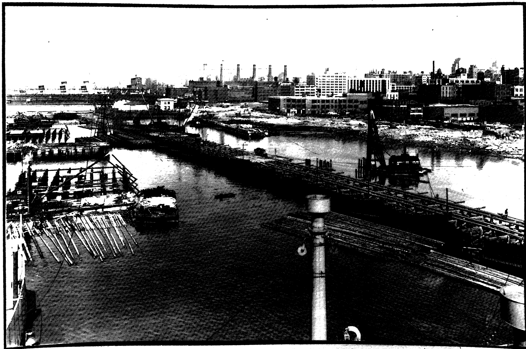
Fig. 61.- Cellular steel sheet-pile cofferdam, 48th St., North River.
