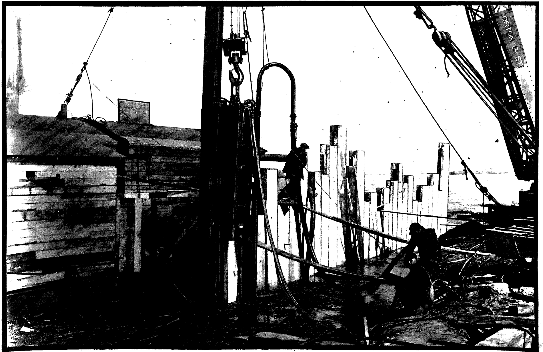
Fig. 46.- Reinforced concrete sheet-piling with steel interlocks.
