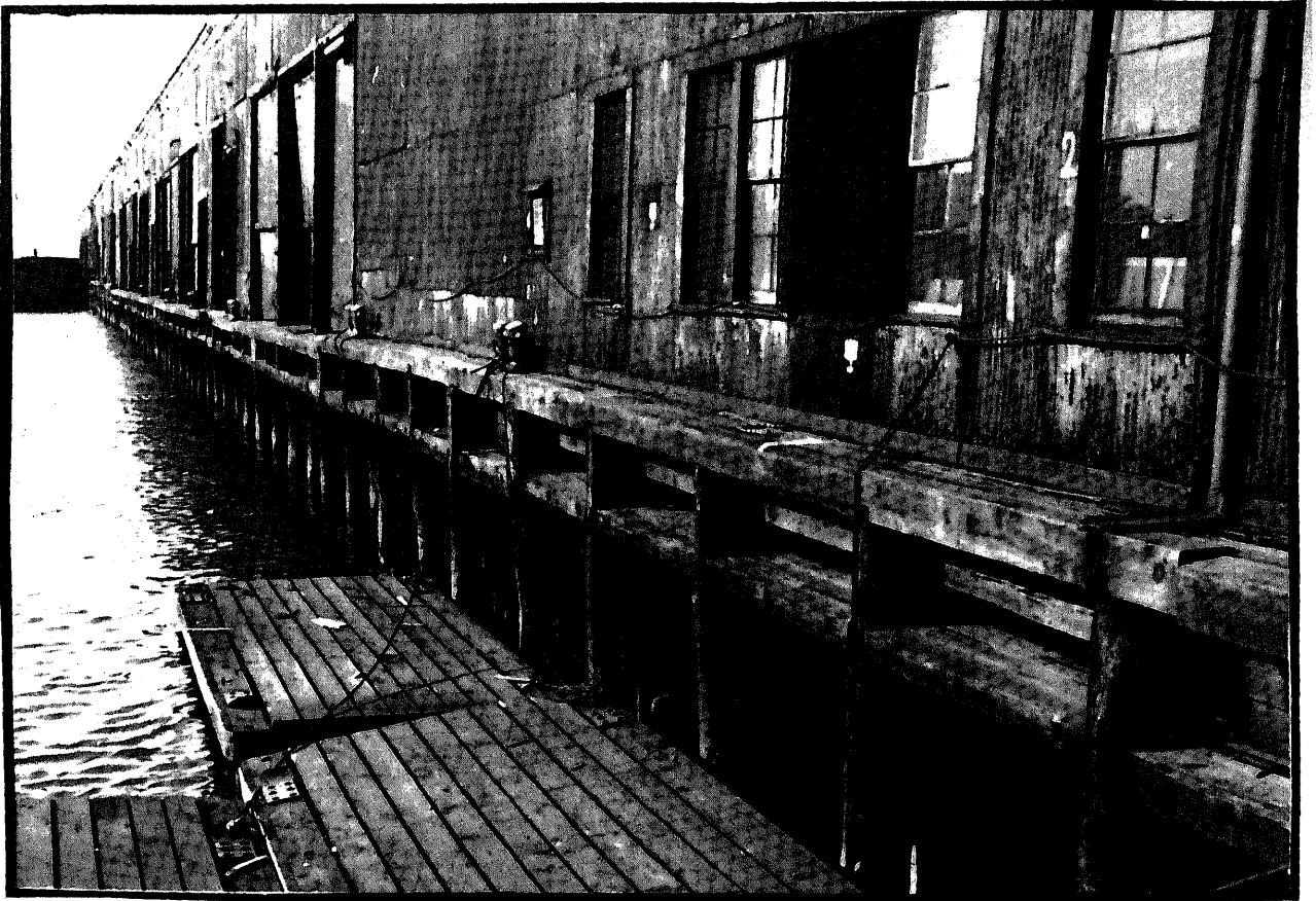
Fig. 49.- Fender piles, cap, and chocks.
