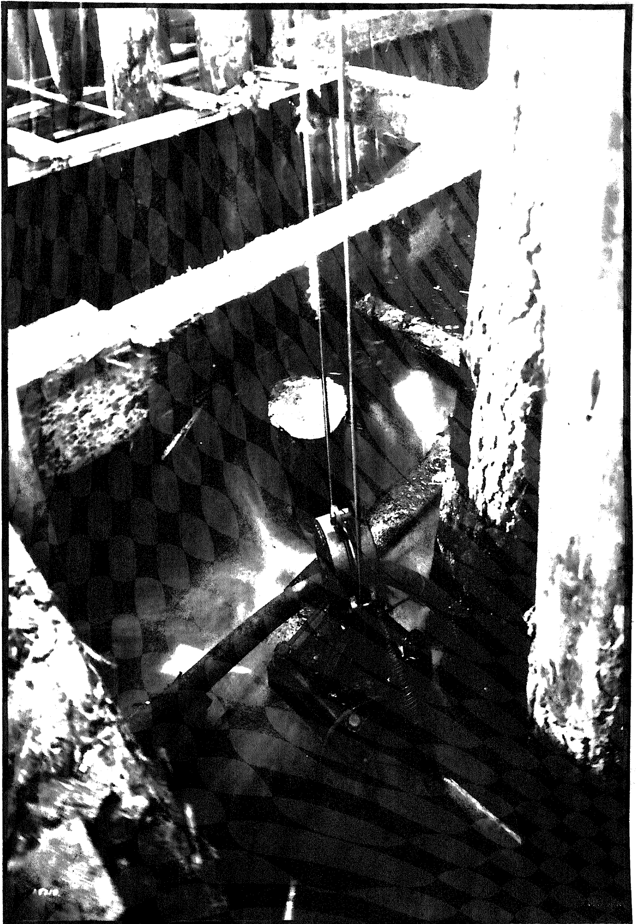
Fig. 77.- Double-acting submarine steam hammer.
