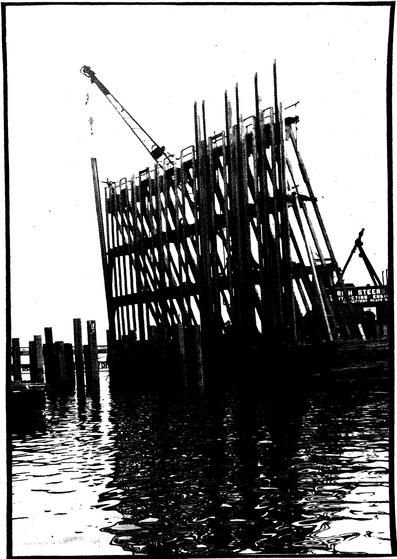
Fig. 35.- Steel H-piles, Seatrain terminal, Edgewater.
