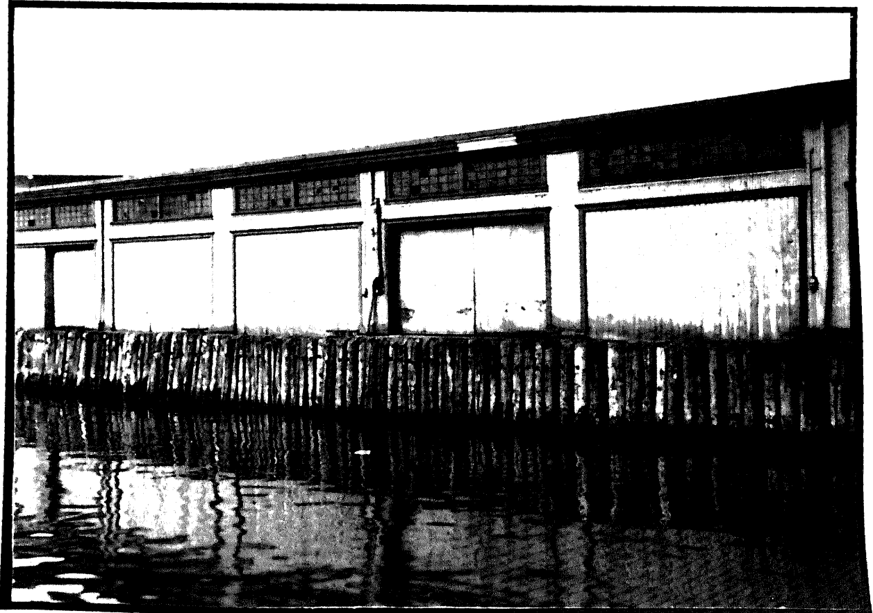
Fig. 50.- Close fender piling.
