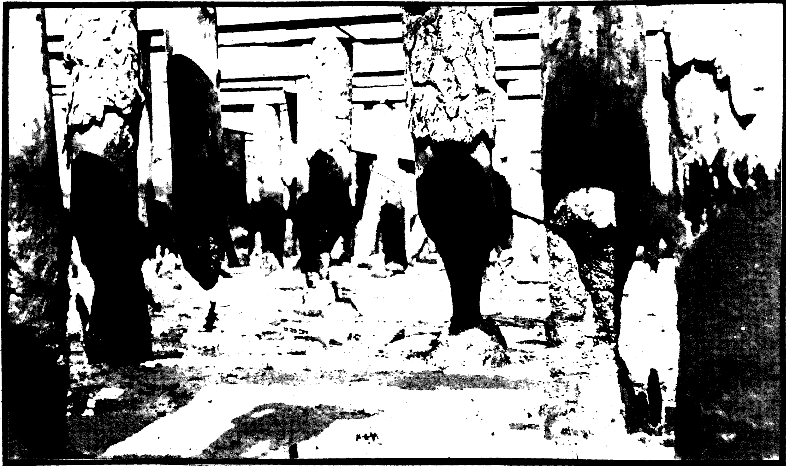
Fig. 65.- Work of marine borers on timber piling.
