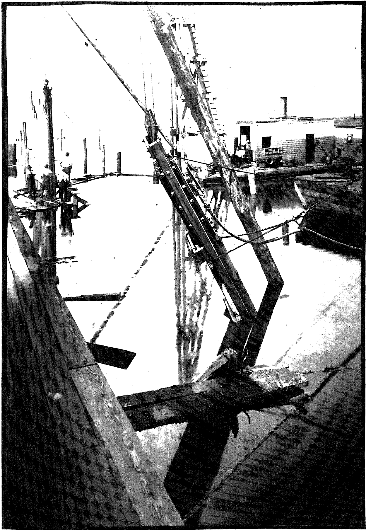
Fig. 83.- Swinging pile leads.
