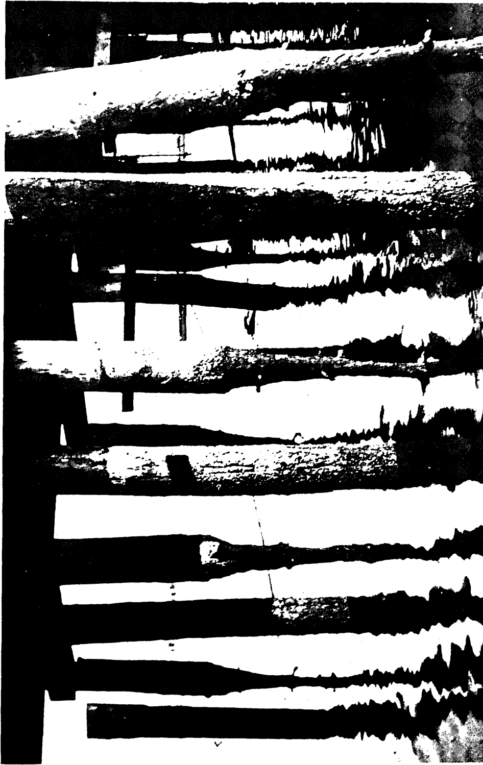
Untreated Douglas fir piling in Oakland Estuary, destroyed by Limnoria . Good piles shown are re-placements.
