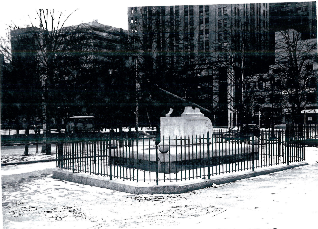
PHOTO 4 OF 46. MILITARY PARK HISTORIC DISTRICT. NEWARK, ESSEX COUNTY, NJ
