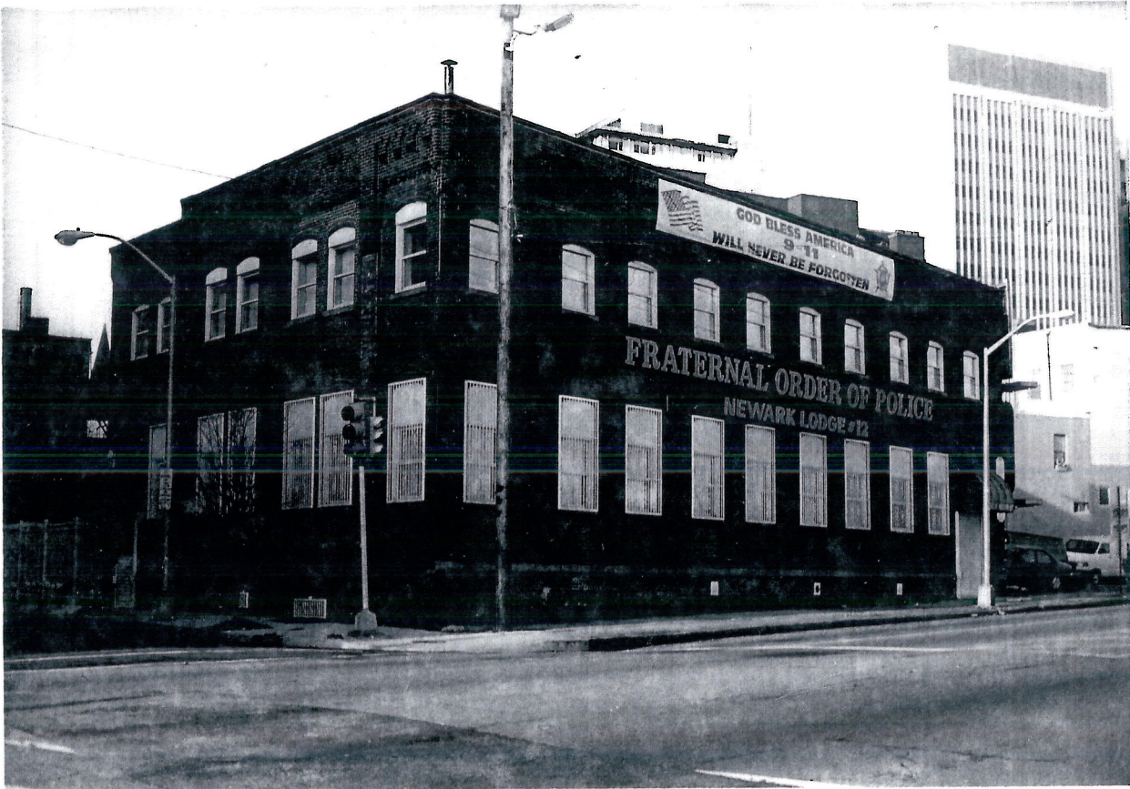
PHOTO 35 OF 46. MILITARY PARK HISTORIC DISTRICT. NEWARK, ESSEX COUNTY, NJ
