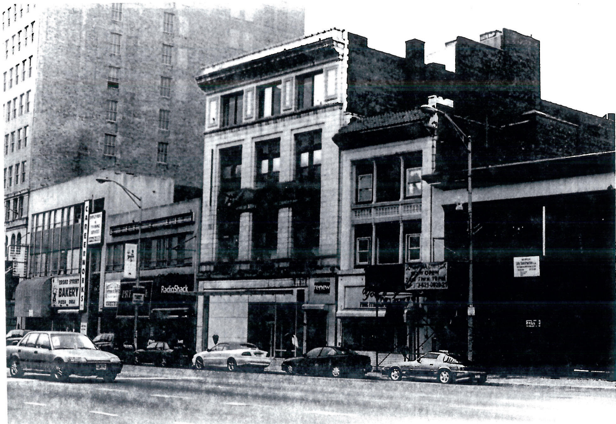
PHOTO 18 OF 46. MILITARY PARK HISTORIC DISTRICT. NEWARK, ESSEX COUNTY, NJ
