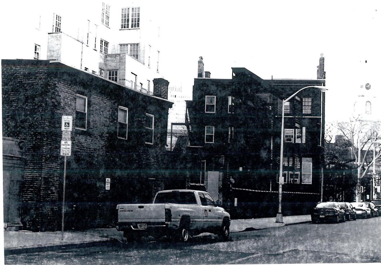
PHOTO 28 OF 46: MILITARY PARK HISTORIC DISTRICT. NEWARK, ESSEX COUNTY, NJ
