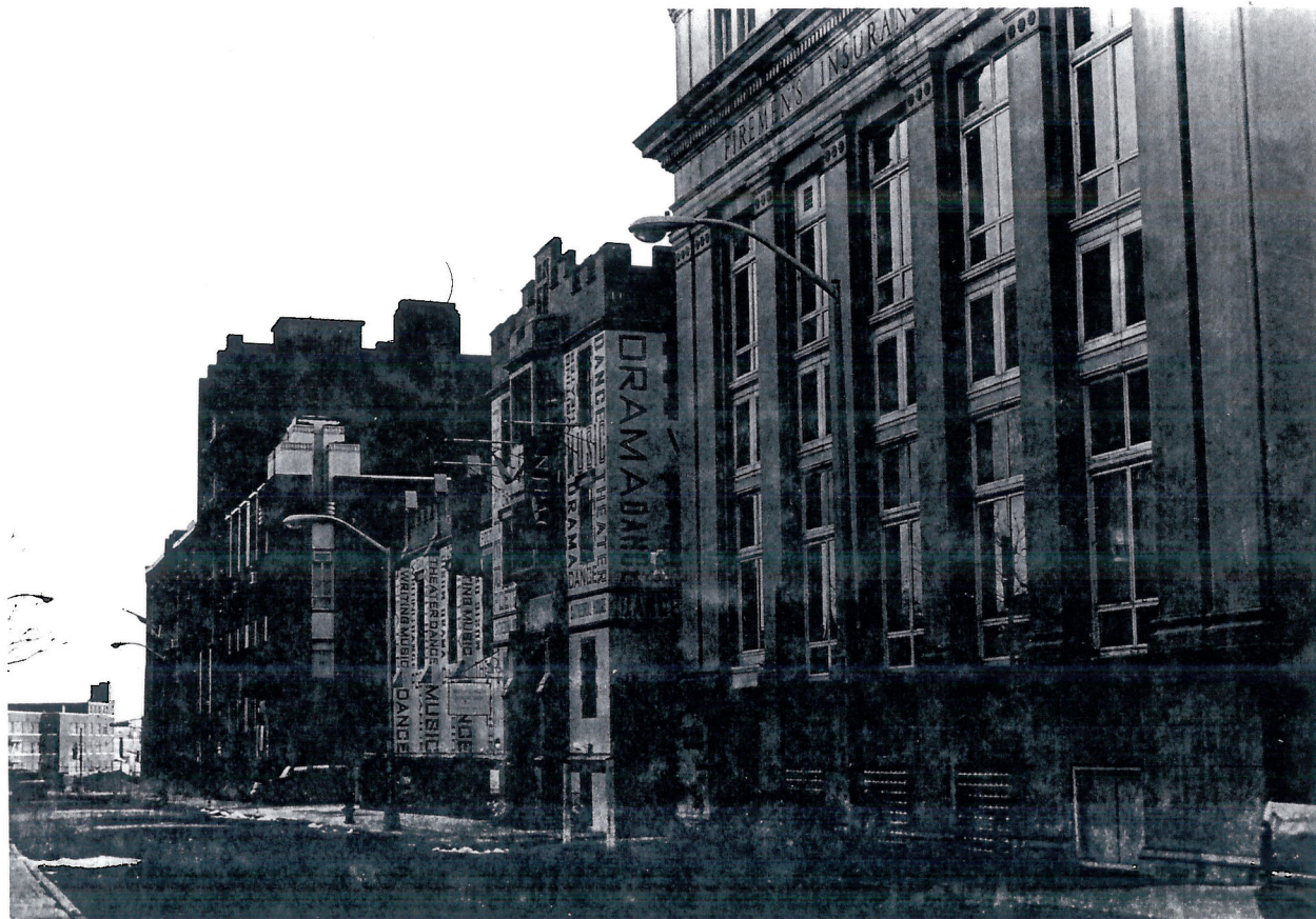
PHOTO 30 OF 46. MILITARY PARK HISTORIC DISTRICT. NEWARK, ESSEX COUNTY, NJ
