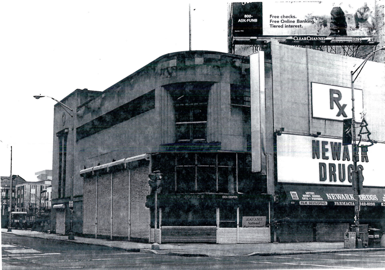
PHOTO 15 OF 46. MILITARY PARK HISTORIC DISTRICT. NEWARK, ESSEX COUNTY, NJ
