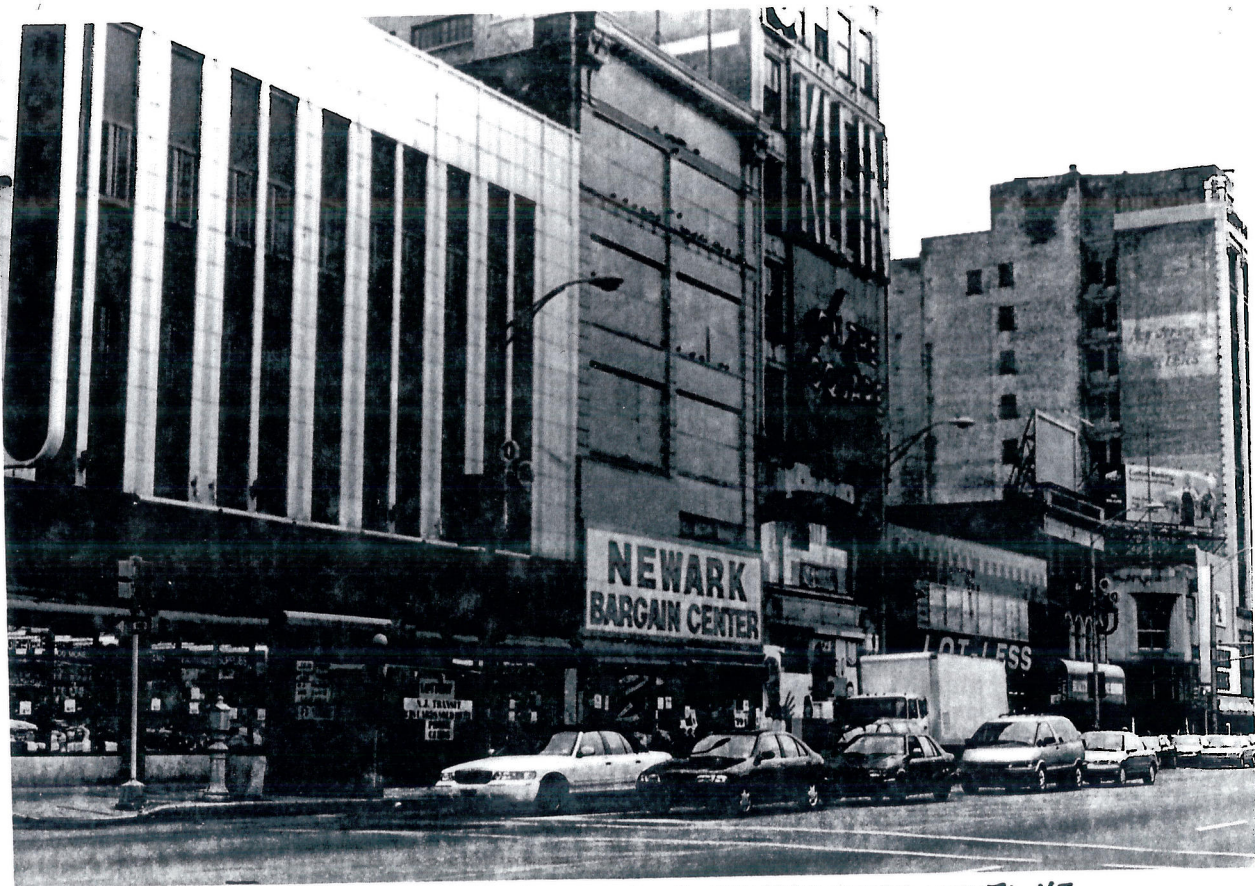
PHOTO 12 OF 46. MILITARY PARK HISTORIC DISTRICT. NEWARK, ESSEX COUNTY, NJ
