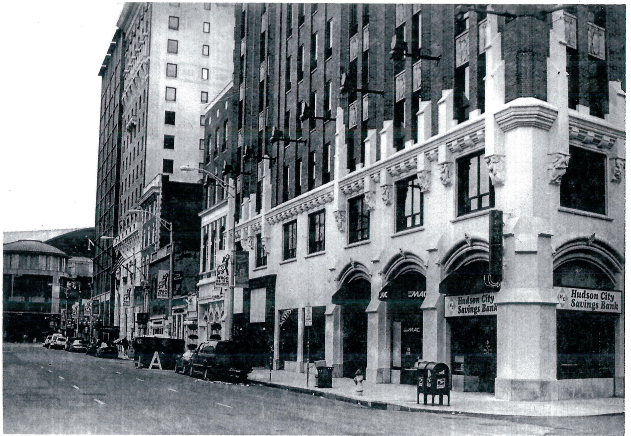
PHOTO 44 OF 46. MILITARY PARK HISTORIC DISTRICT. NEWARK, ESSEX COUNTY, NJ
