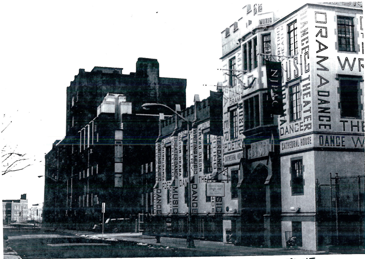
PHOTO 33 OF 46. MILITARY PARK HISTORIC DISTRICT. NEWARK, ESSEX COUNTY, NJ
