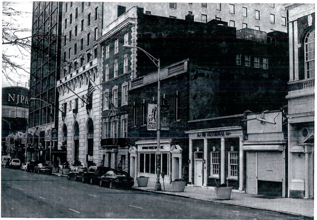
PHOTO 43 OF 46. MILITARY PARK HISTORIC DISTRICT. NEWARK, ESSEX COUNTY, NJ
