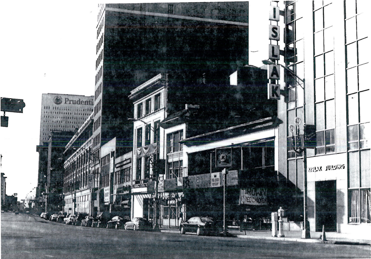
PHOTO 19 OF 46. MILITARY PARK HISTORIC DISTRICT. NEWARK, ESSEX COUNTY, NJ
