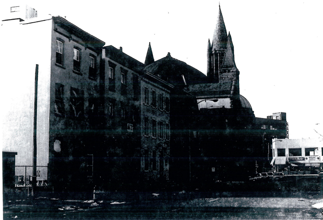
PHOTO 38 OF 46. MILITARY PARK HISTORIC DISTRICT. NEWARK, ESSEX COUNTY, NJ
