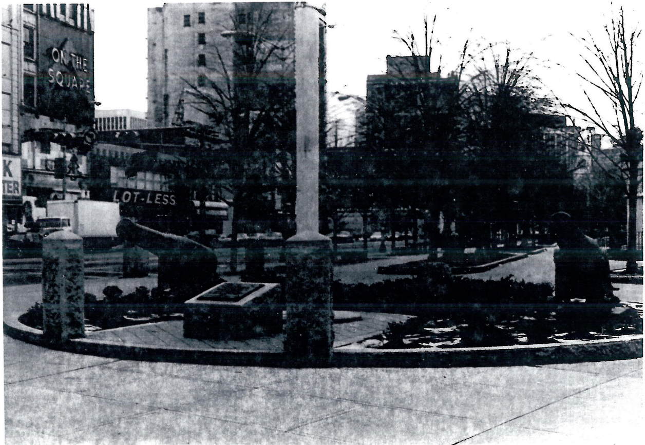
PHOTO 6 OF 46. MILITARY PARK HISTORIC DISTRICT. NEWARK. ESSEX COUNTY, NJ
