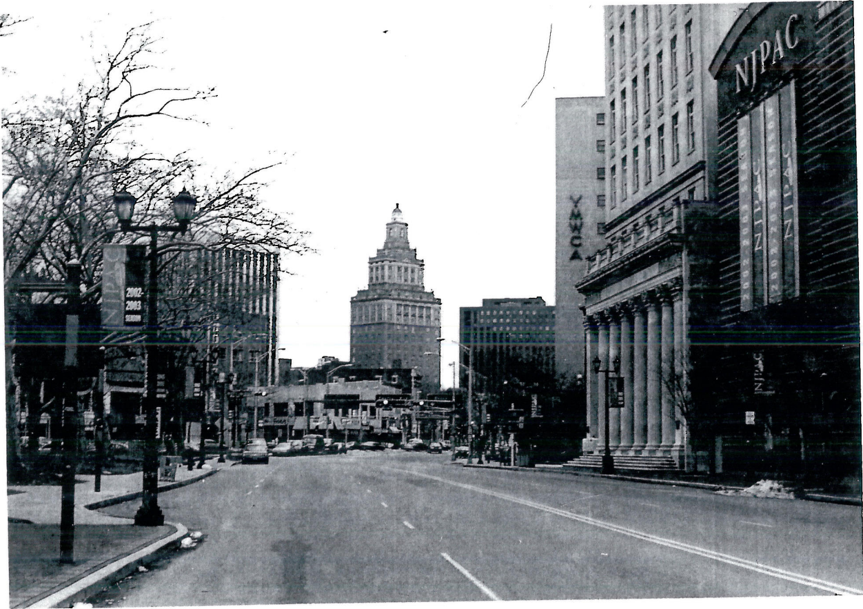
PHOTO 41 OF 46. MILITARY PARK HISTORIC DISTRICT. NEWARK, ESSEX COUNTY, NJ
