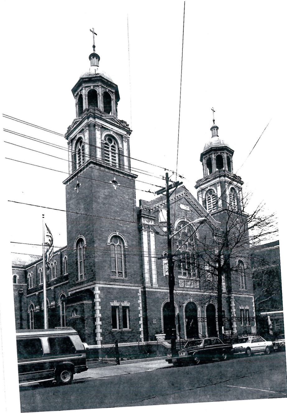
Photo 3 of 18: Pulaski Street facade. View looking southeast.
