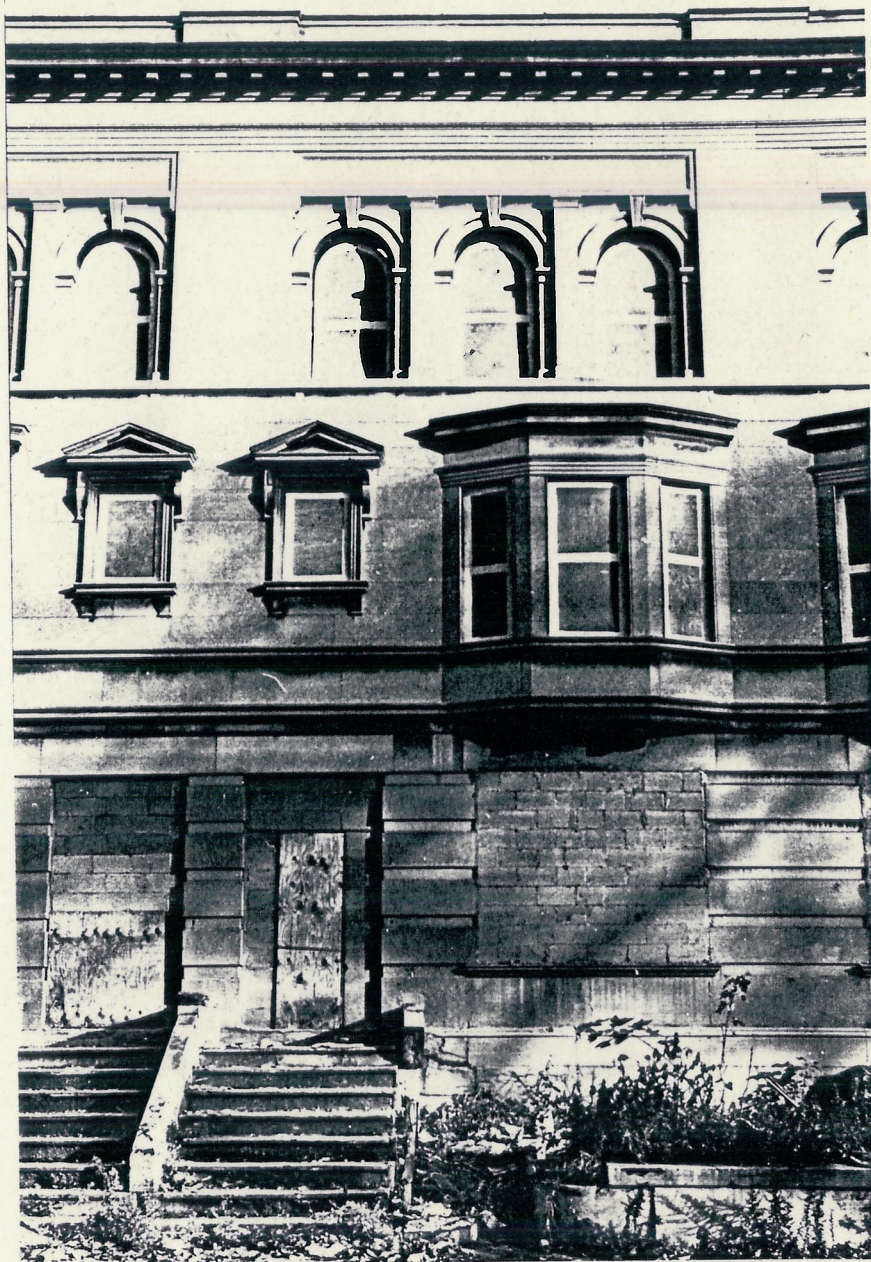
Photo 7. 142 Broad Street, looking east
