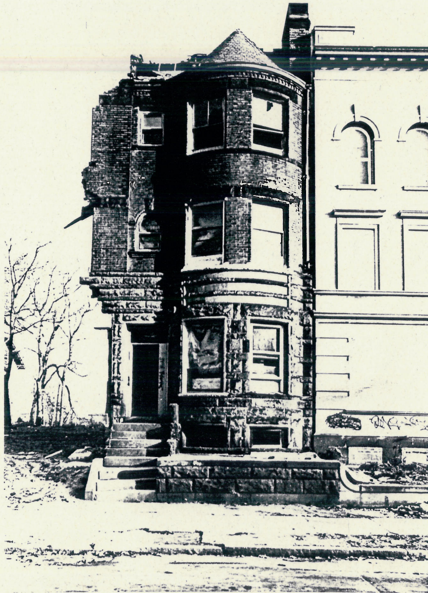
Photo 4. 136 Broad Street, looking east
