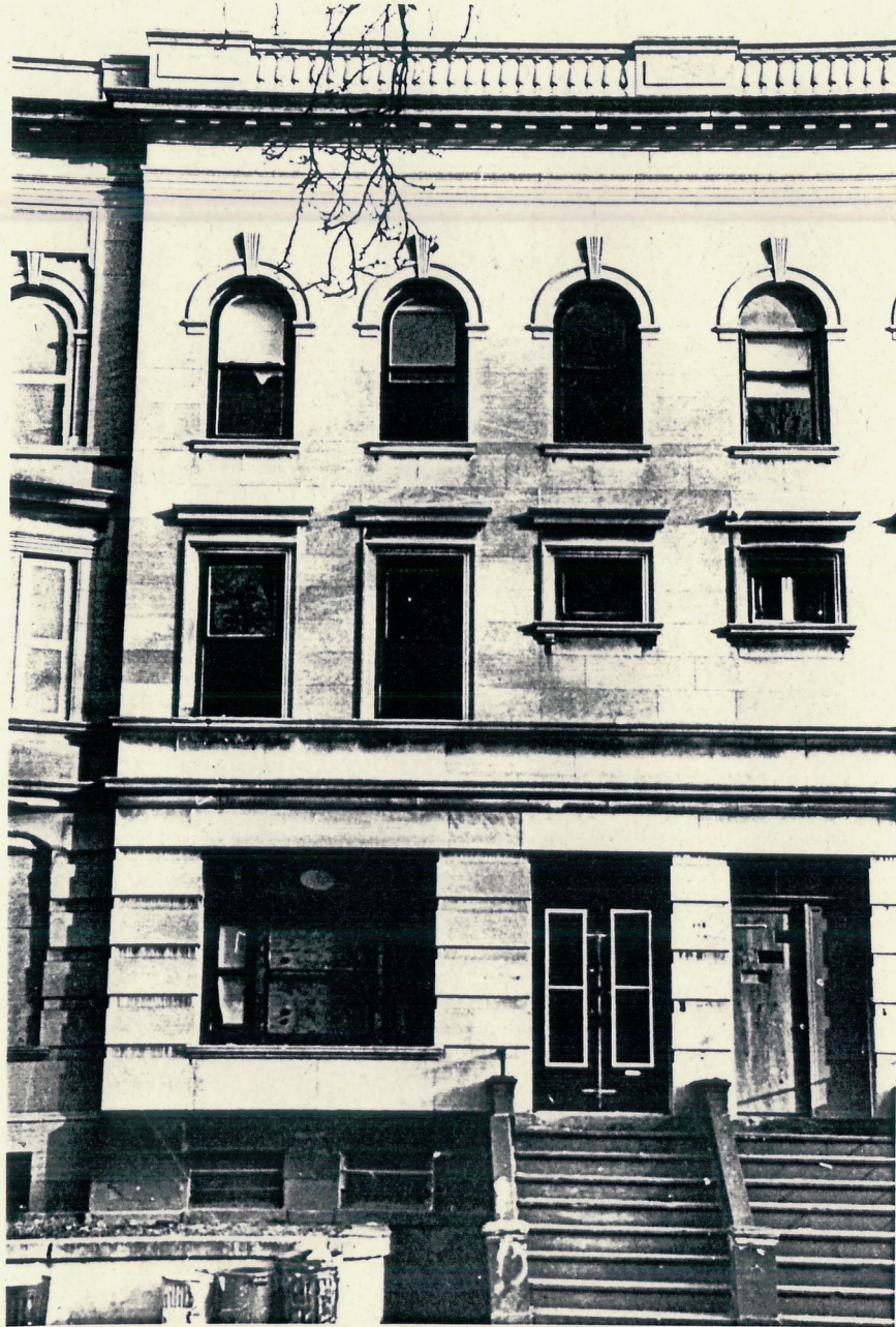
Photo 10. 146 Broad Street, looking east
