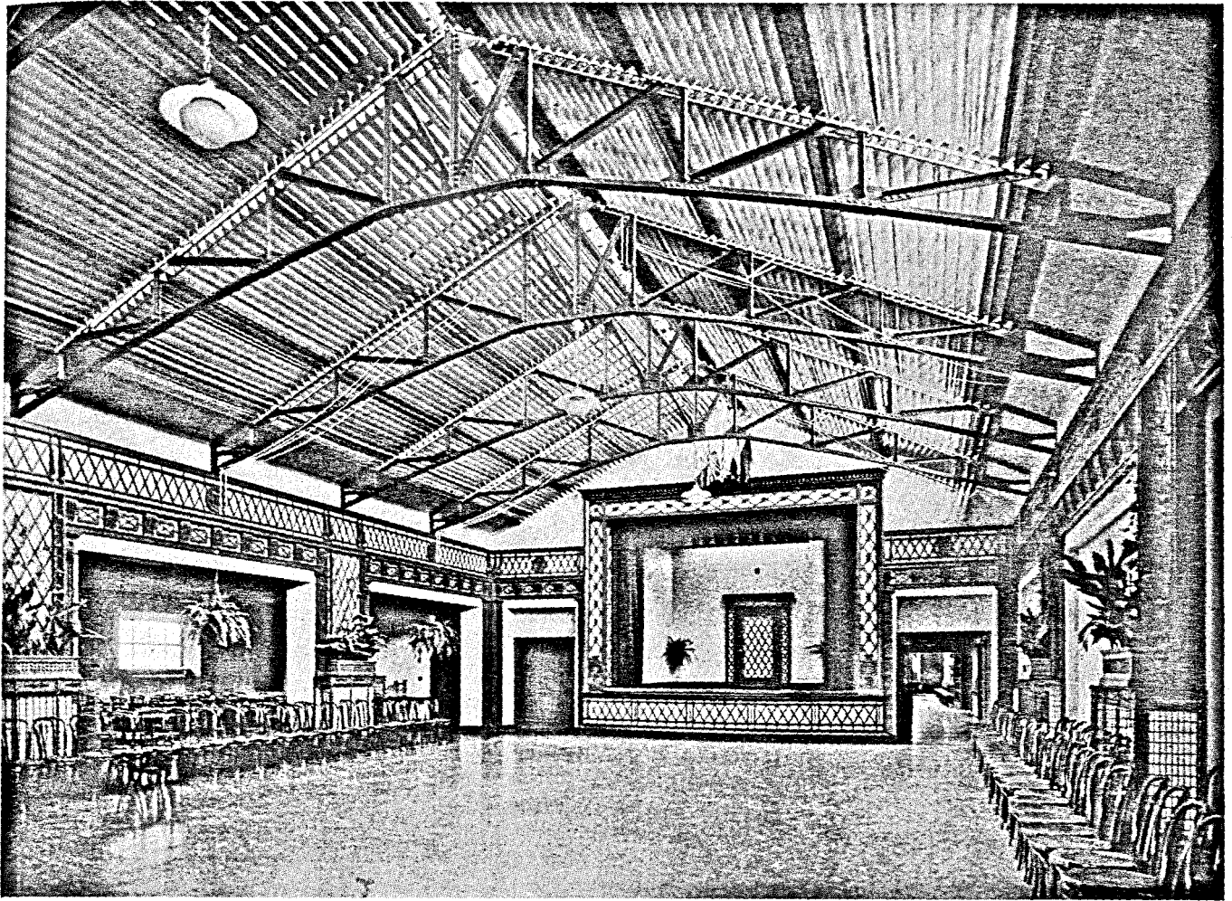
AUDITORIUM, SIXTH FLOOR.
